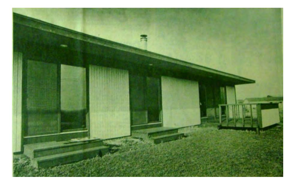
Lo Cal House - USA – 1976 Wayne Shick and Bud Konzo R-30 double stud walls R-30 vented roof Triple glazed windows Air to air heat exchanger
