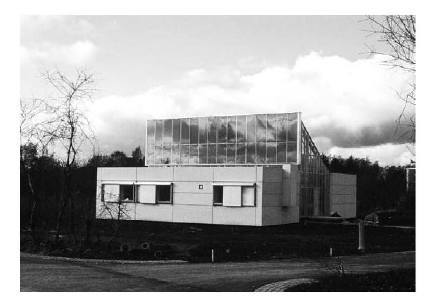
Lyngby House - Denmark – 1975 Null-Energi-Haus Vagn Korsgaard – Technical University of Denmark Double walls, R-40 walls, R-60 roof Air to air heat exchanger Double glazed windows with insulating shutters Solar thermal – 8,000 gal storage tank
