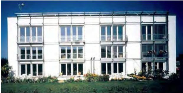
Passivhaus – Darmstadt - Kranichstein – 1991 Super Insulated Air tight Air to air heat exchanger Subsoil heat exchanger
