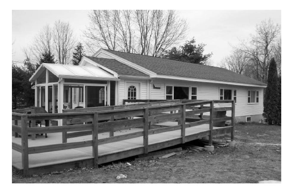
Leger House - USA – 1977 Double wall – R 40 walls R 60 ceiling Airtight construction Air to air heat exchanger
