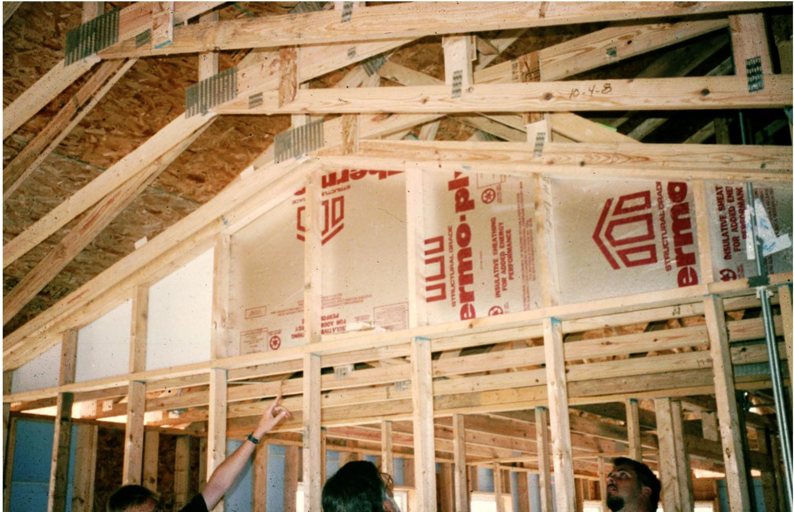
Tall 2x6 walls bow outwards during the winter...due to the temperature difference leading to a relative humidity difference...
