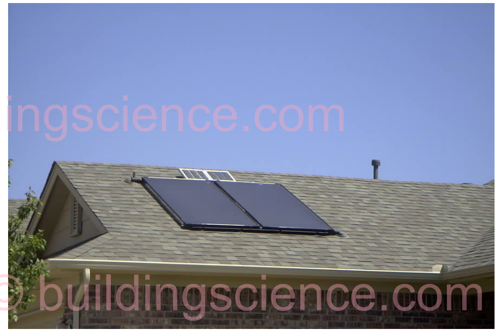
Panels on south roof
