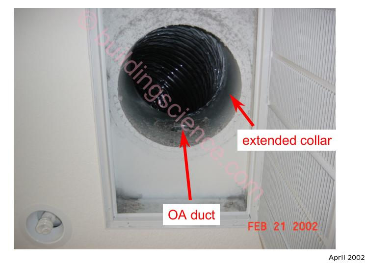
**Central-fan-integrated supply ventilation** Unvented-cathedralized attic configuration With motorized damper and damper cycling control
