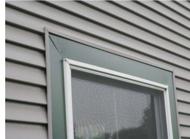
Existing window trim - head
