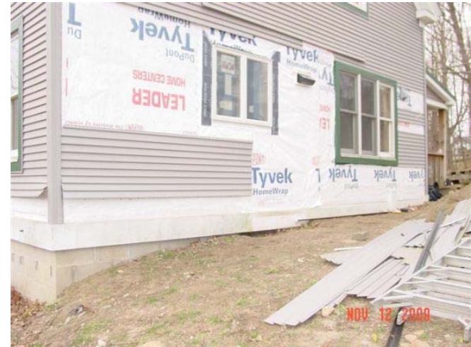
Siding removed to remediate flashing
