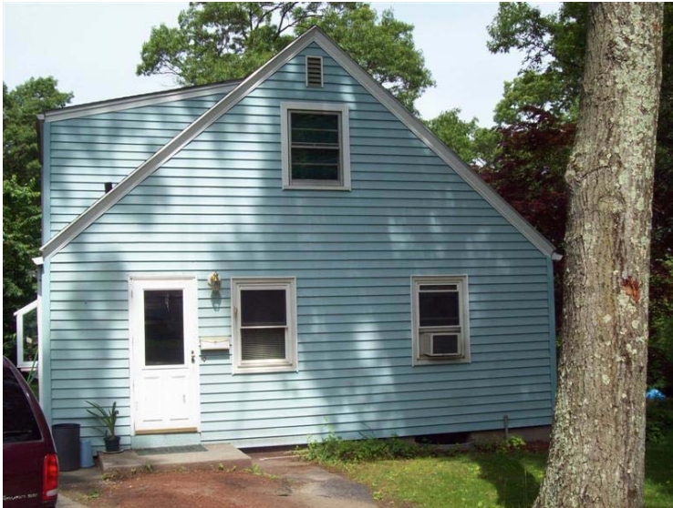
Tweedly residence pre-retrofit
