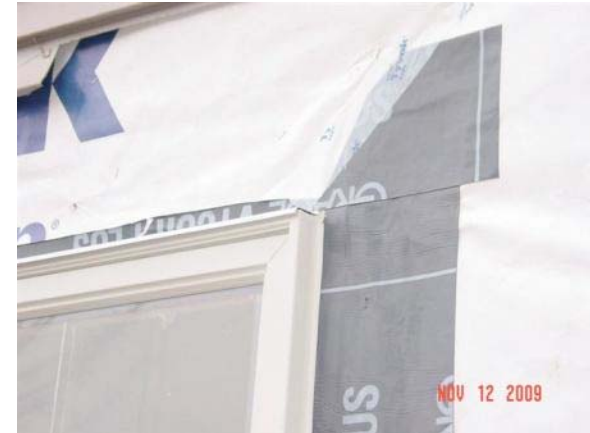
Head flashing at new window
