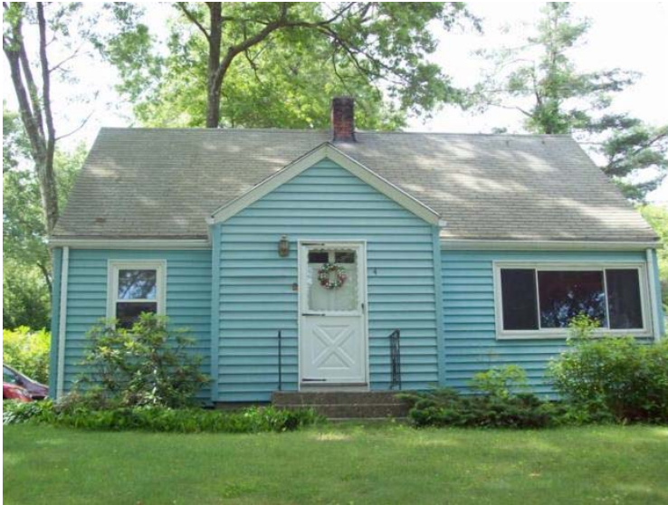
Tweedly residence pre-retrofit
