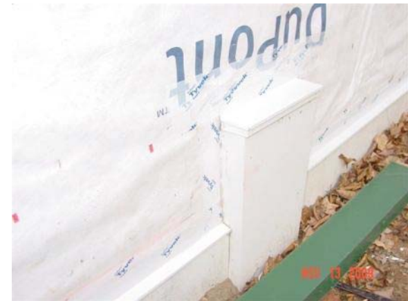
Drainage plane remediation at base of wall
