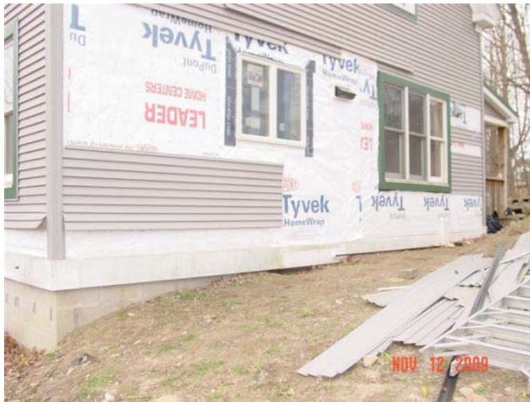
Siding removed to remediate flashing
