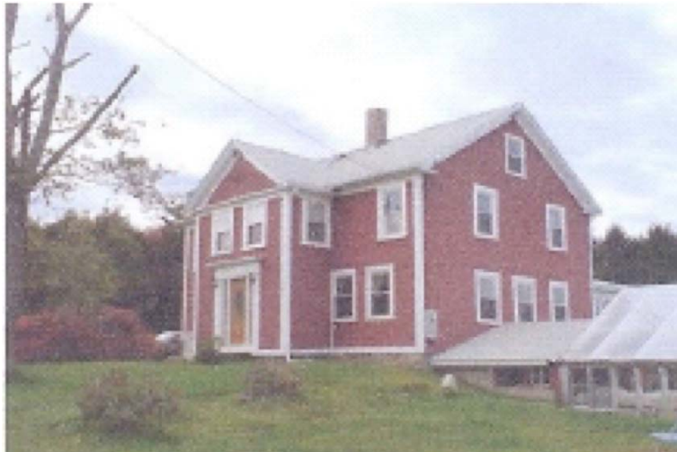
Red House Farm pre-retrofit
