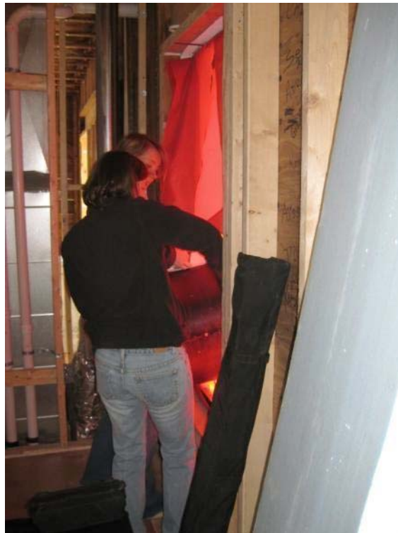
Blower door fan installed in window
