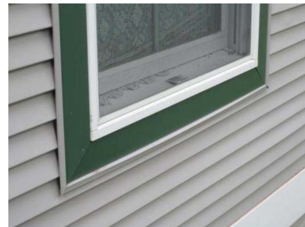
Existing window trim - sill
