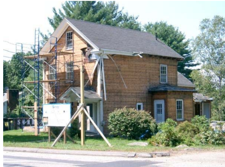
Bedford Farmhouse during demolition
