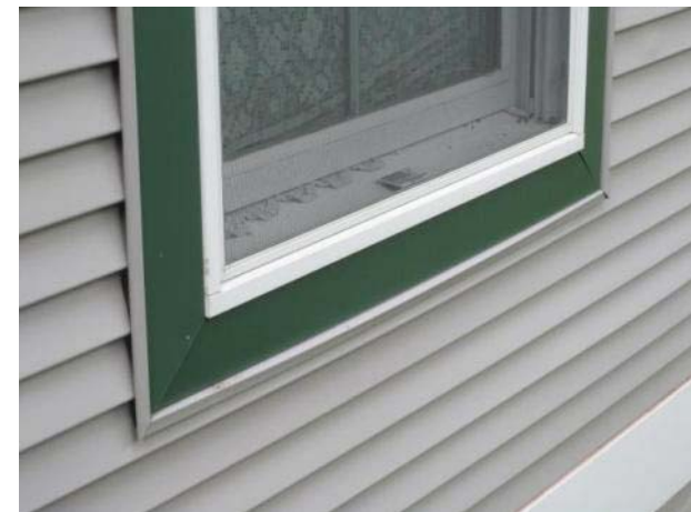
Existing window trim - sill
