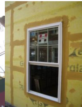
Airflow Control No. 28/79
