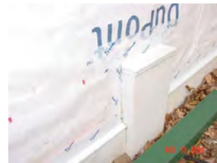
Drainage plane remediation at base of wall
