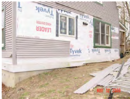
Siding removed to remediate flashing
