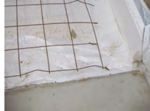
EPS under slab with polyethylene
