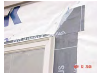
Head flashing at new window
