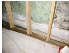
EPS under slab with polyethylene
