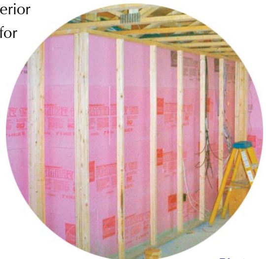
Photograph 1 XPS against basement wall with framed wall
