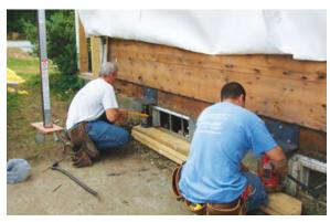
Lifting a sill to insert a capillary break
