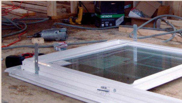
Photograph 6: Window Attachment —Typical flanged residential windows are installed with the flanges overlapping the exterior surface of the rigid foam insulating sheathing. Attachment is with mounting straps typically used with masonry openings.
