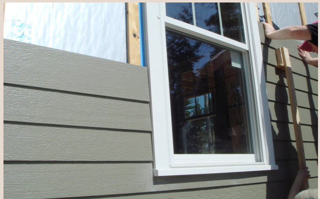
Photograph 7: Exterior Window Trim —Exterior trim is attached over the top of the exterior 1x4 wood furring. Standard water management (pan flashing and flashing tape) for rigid foam sheathing is used.
