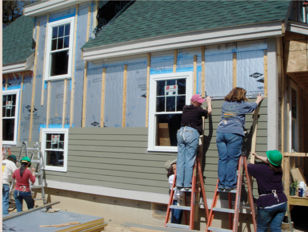
Photograph 4: Cladding Attachment —Standard cladding attachment is used to attach cladding to the 1x4 wood furring. Published tables for cladding attachment found in the model building codes is followed.
