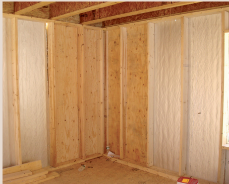
Photograph 2: Advanced Framing —2x6 studs on 24 inch centers, stack framed, single top plates, two stud corners, no jacks, no cripples. Almost 40 percent of the framing elements typical in traditional wood frame construction have been removed. The framing factor is reduced from 25 percent to less than 15 percent. The exterior sheathing was foam board insulation; racking resistance was provided at corners by structural sheathing.
