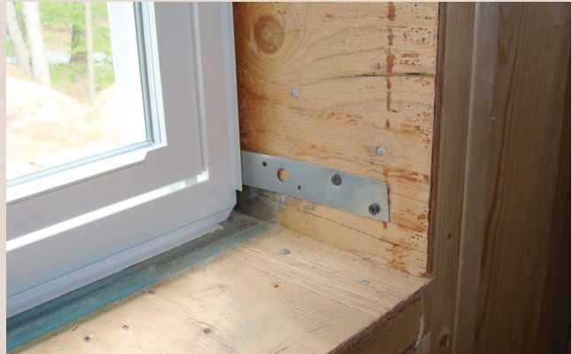
Photograph 5: Window Openings —Openings were lined with ½ inch thick plywood “boxes” that extended outward 4 inches past the exterior face of the stud wall framing such that their exterior edge lined up “flush” with the exterior surface of the exterior rigid foam insulating sheathing.
