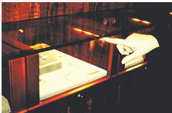
Photograph 3: Display Cabinets —Each cabinet “compartment” has a display light. The individual lights generate heat – enough to warm each case compartment to about 140 degrees. The working hypothesis is that the lights generate enough heat to cause the cabinetry to smell. The cabinetry is some kind of “was-wood-once” composite with a “who-knows-what” finish.
