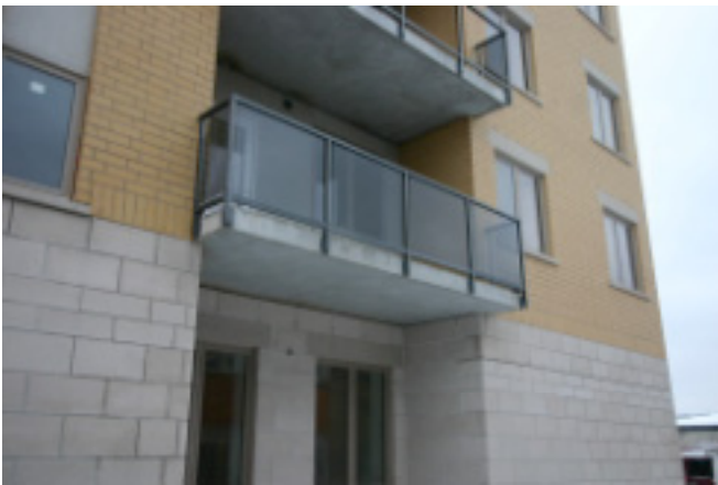
Photo 8: Balcony Offset Point Supports. Precast balcony supported intermittently to break thermal bridge.
