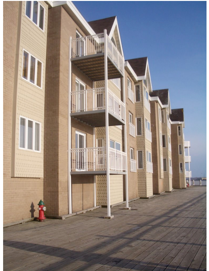
Photo 11: Stand-Alone Balcony. Balconies have their own structural frame and foundation.
