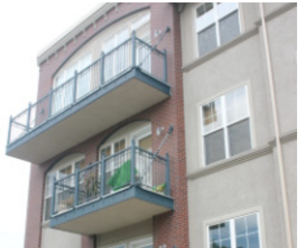
Photo 10: Hang in There. Offset point supports combined with tie rods.
