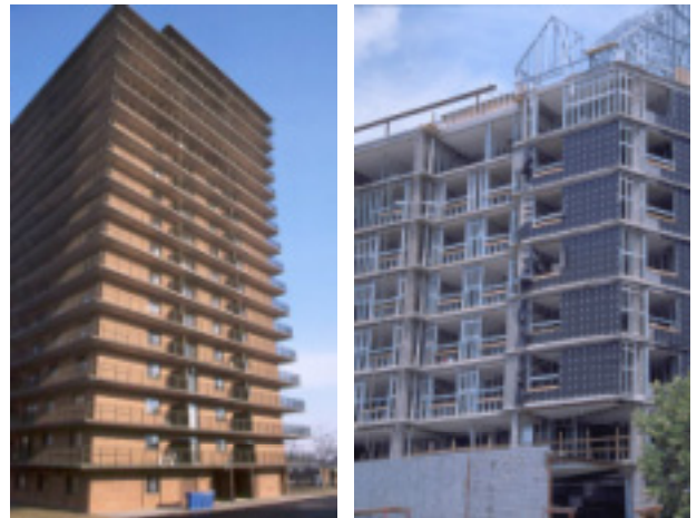
Photo 1 (left): “Harley Davidson” Architecture. The projecting concrete slabs transfer heat across the enclosure.
