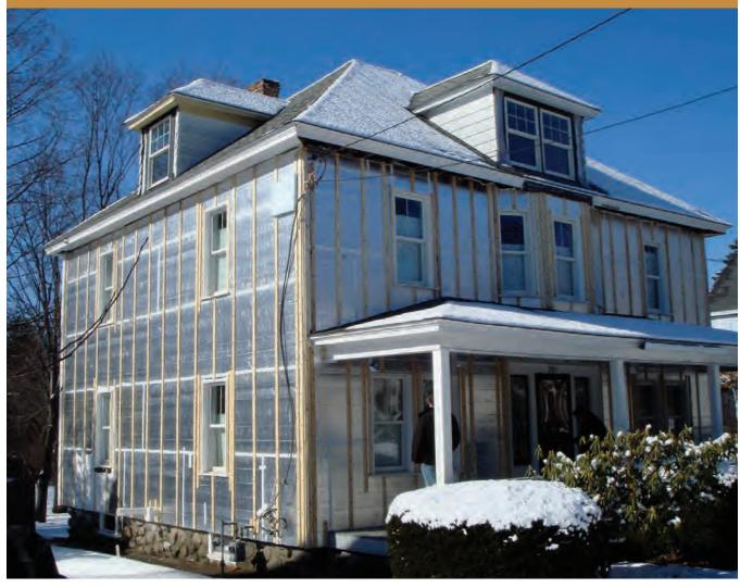
incident water drains to the outside. The ¾-in. ventilated space provides added protection (water is not "sand wiched" between the clapboard and the underlying structure, plus the space allows for ventilation drying).
