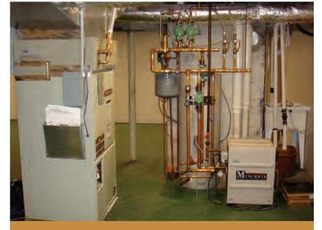
Mechanical systems upgrades in the basement include an air handler, high efficiency boiler and a super insulated water tank.
