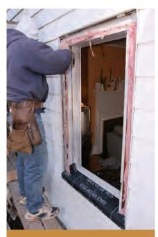
Insulation was installed around the window opening. The membrane pan flashing installed to receive the replacement windows was extended upwards and wrapped the entire opening.
