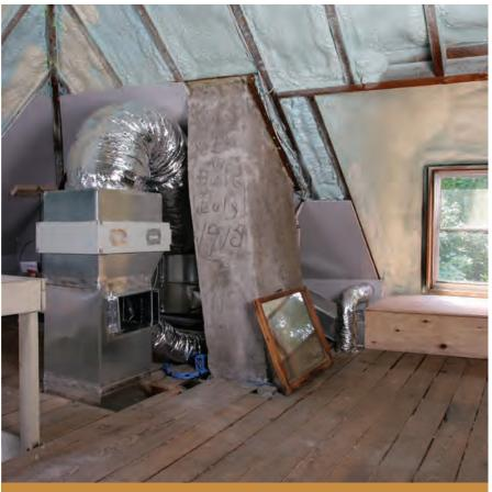
An air handler in the attic supplies the attic and second floor. A pleated media filter was installed at the return. The original builders left their mark embedded in the parge coat over the chimney, "Built July 1915."
