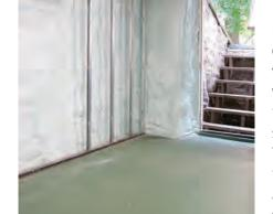
Exposed spray foam insulation on the basement walls was covered with gypsum board over metal studs.
