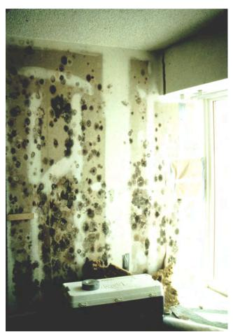
Photograph 2: Vinyl wall covering removed to expose mold on hotel room wall
