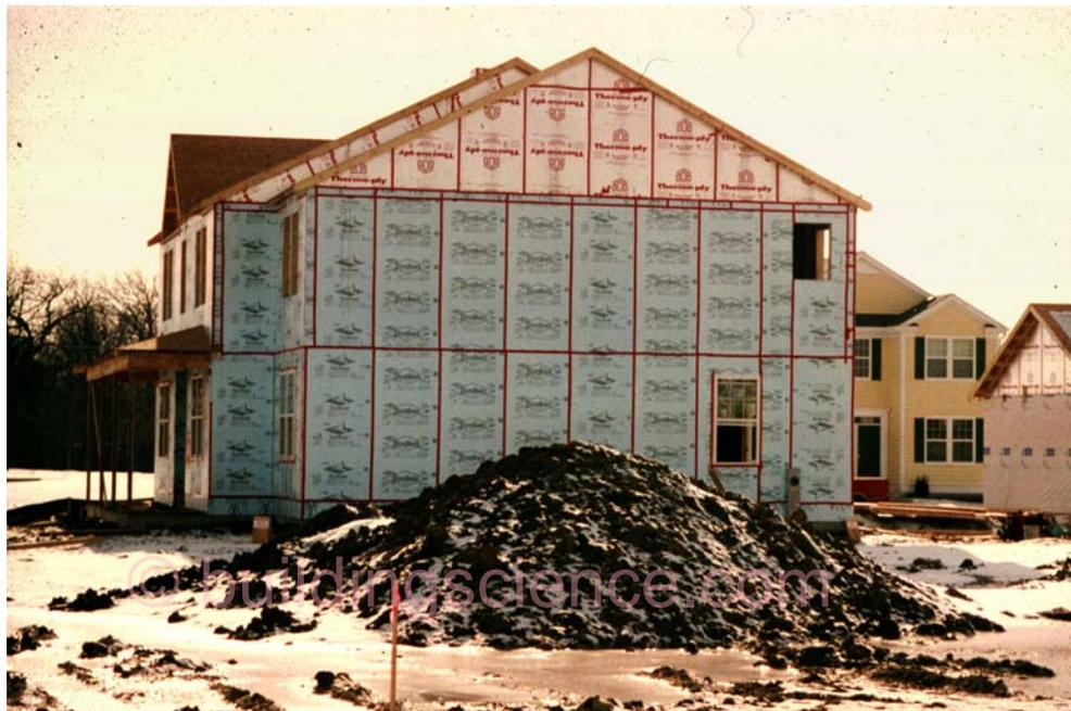
Photograph 3: Rigid foam insulating sheathing drainage plane
