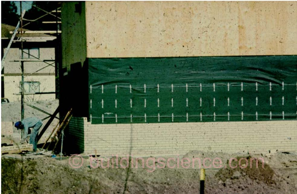
Photograph 1: Tar paper or building paper drainage plane
