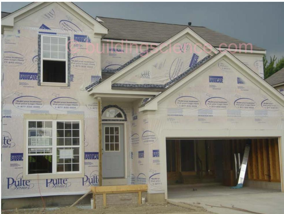
Photograph 2: "Housewrap" drainage plane
