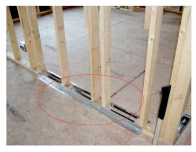
Unsealed wall cavities used as return air plenum
