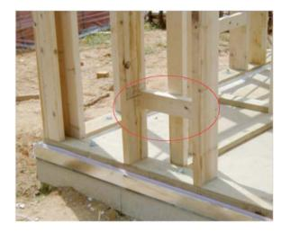
Ladder blocking should have been used at the interior wall at exterior wall connection
