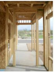
Excessive framing in a non-load bearing wall above a sliding glass door (above left), in a non-load bearing door opening (above right), in a non-load bearing wall above a window (below left) and in a non-load bearing wall above a bay window (below right)
