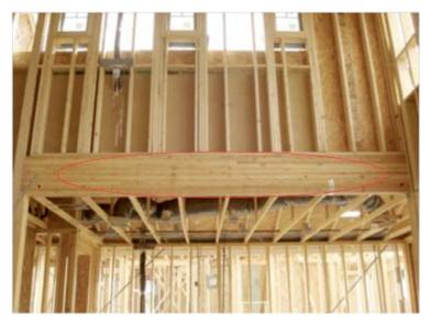
Interior framed beam; note the cripple studs are not required above the beam/below the windows
