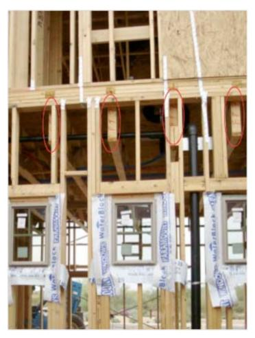
• A top chord bearing truss is used to support the second story floor assembly; the ends of these trusses are visible on the exterior.
