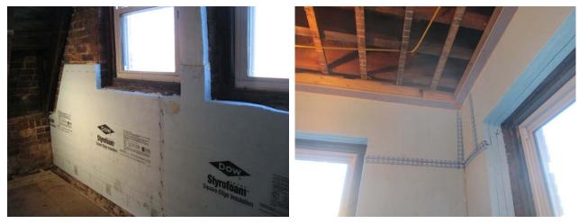
Figure 18: Installation of foam on masonry (left); Multiple layers of insulation (right)
