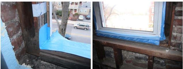
Figure 19: Openings properly flashed (left); Window re-installed (right)
