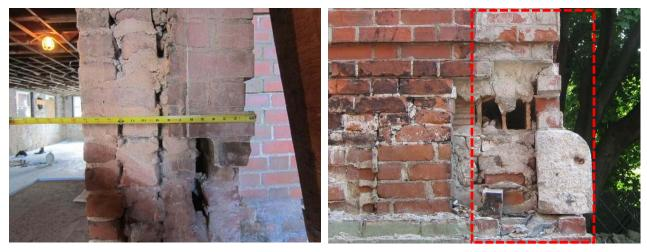
Figure 6: Wall section at solid brick (left) and at hollow clay block infill (right) conditions
