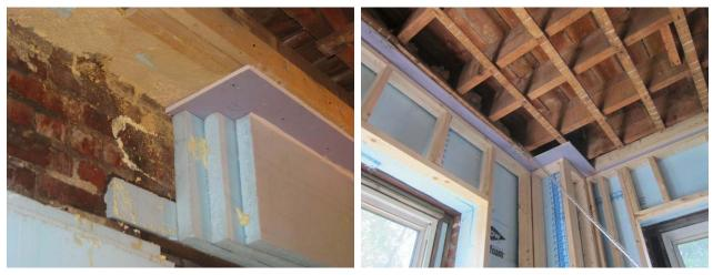
Figure 20: Floor/ceiling fire separation gypsum board (left); Conditions after interior framing (right)
