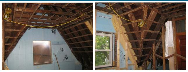
Figure 22: Rigid wall insulation left clear of roof (left) and infill with spray foam (right)
