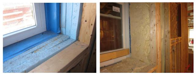
Figure 21: Rigid wall insulation around window (left) and infill with spray foam (right)
