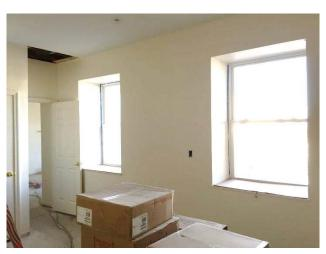
Figure 25: Gypsum Board installed
