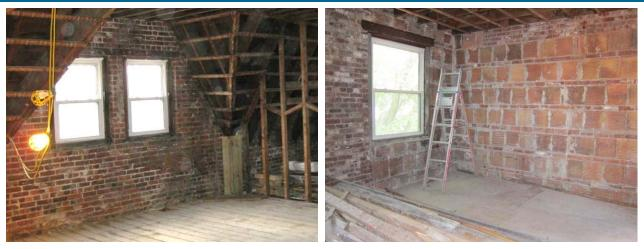
Figure 5: Exterior wall conditions at solid brick (left) and hollow clay block infill (right) conditions
