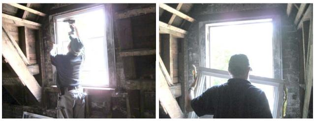
Figure 16: Removal of existing window (left) and window removed (right)
