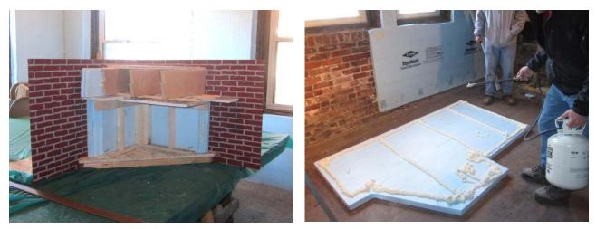
Figure 17: Mockup (left); Use of polyurethane adhesive (right)
