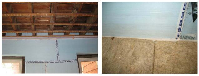
Figure 23: Rim joist foam blocks (left); air seal between rigid foam and floor (right)
