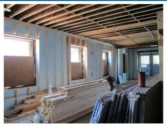
Figure 24: Framing installed inboard of insulation
