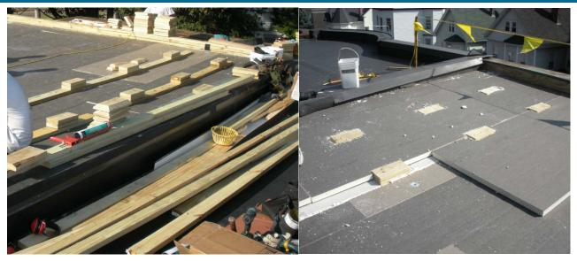
Figure 19: Blocking for future PV installation
