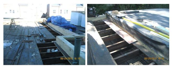
Figure 14: Existing boards removed near roof perimeter with P.T. plywood installed at parapet (left); strip of OSB sheathing with integrated water resistive barrier at parapet (right)
