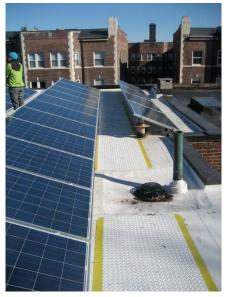
Figure 20: Roof membrane with blocking for PV system rack (left); finished roof (right)
