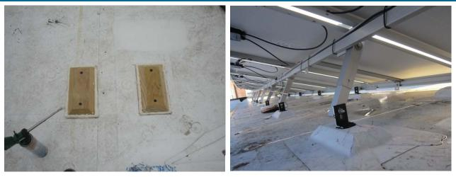
Figure 21: PV system rack attachment during construction (left) and completed (right)
