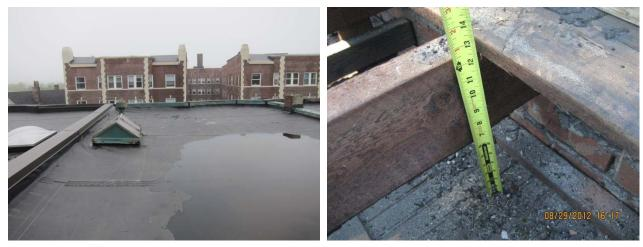
Figure 13: Existing roof cladding to be removed (left) and verification of existing conditions (right)
