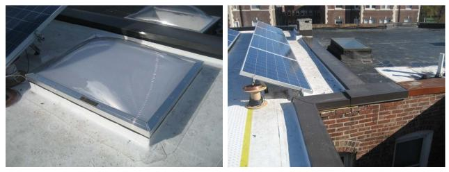
Figure 22: Skylight installation (left) and metal cap flashing (right)
