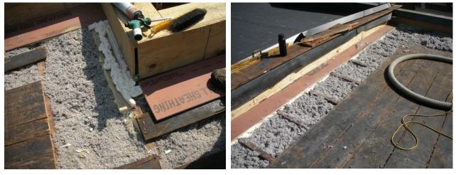
Figure 16: Fibrous insulation installed in the rafter cavity with air sealing details
