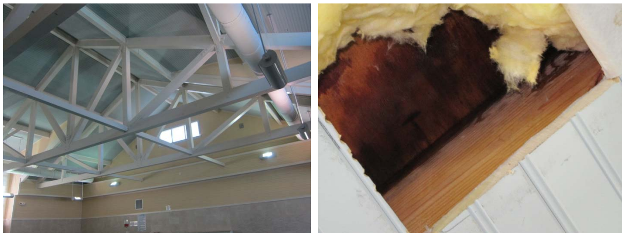
Figure 89: Ridge condensation issues; Zone 3A pool with interior polyethylene vapor barrier
