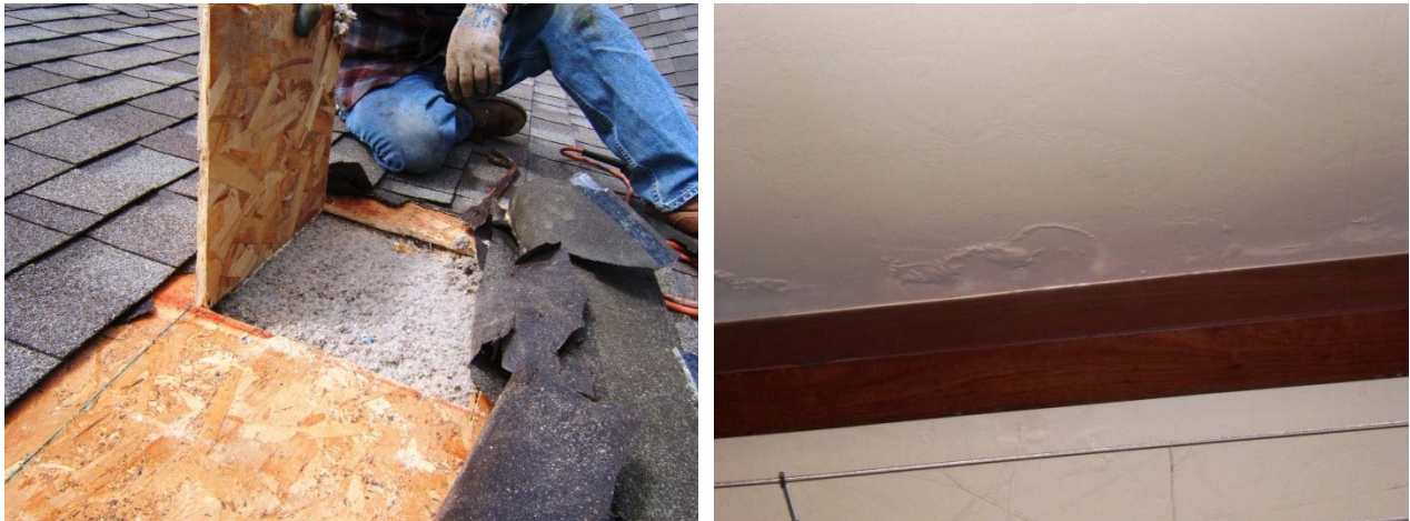
Figure 10: Dry sheathing lower at roof (L), and interior ridge conditions (R)
