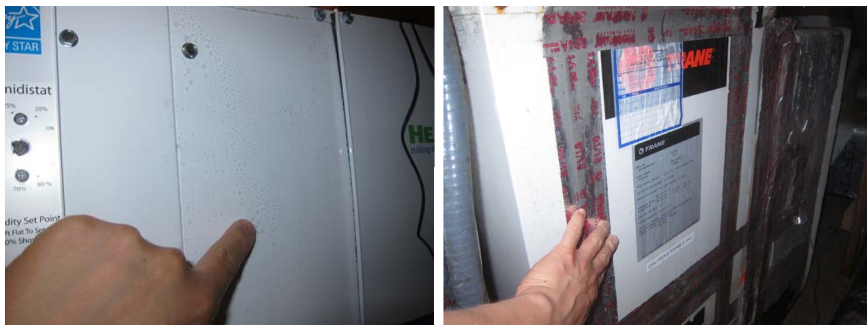
Figure 3: Condensation on HVAC equipment located in vented attic (Zone 2A)
