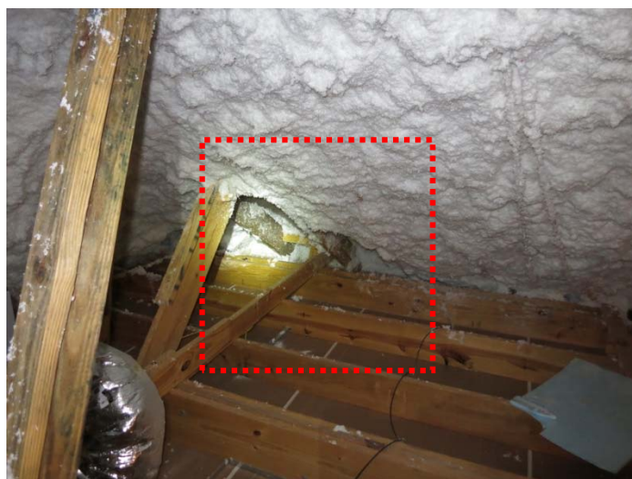
Figure 108: Air leakage at roof-to-wall details at dormer/intersecting roofs (Location A)
