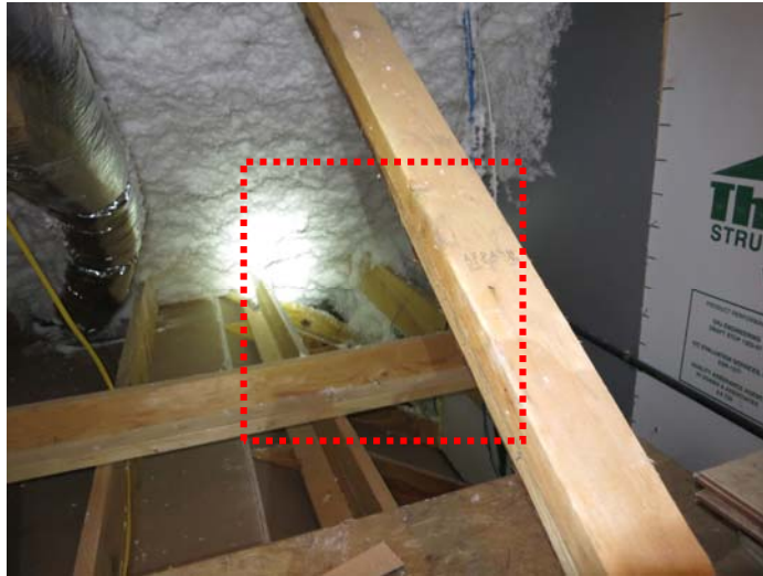
Figure 111: Air leakage at roof-to-wall details at roof-wall intersection (Location C)
