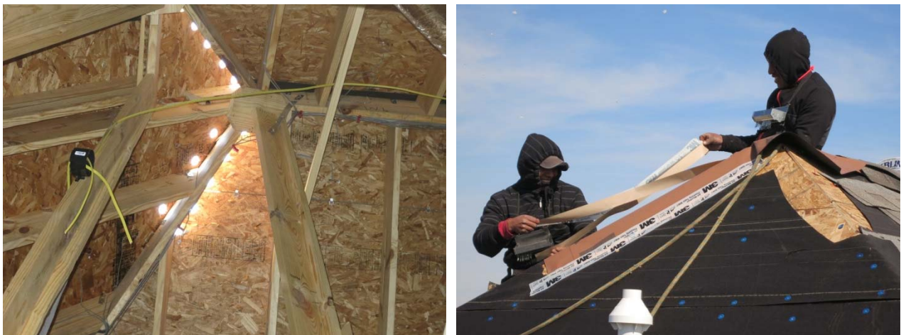
Figure 97: Hip “diffusion port” drilled hole detail (L); permeable membrane applied at hips
