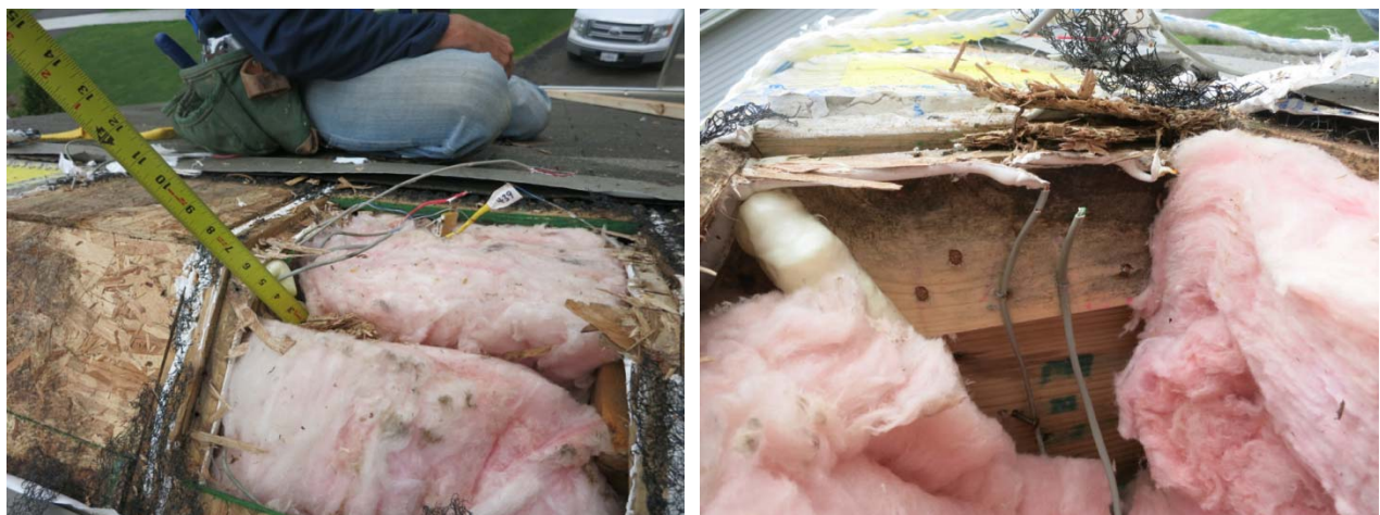
Figure 76: Fiberglass batt and framing conditions at ridge, Roof 4 (L) and Roof 5 (R)
