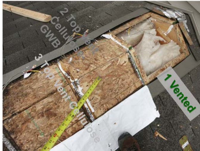
Figure 69: Ridge sheathing conditions, Roofs 1, 2, and 3
