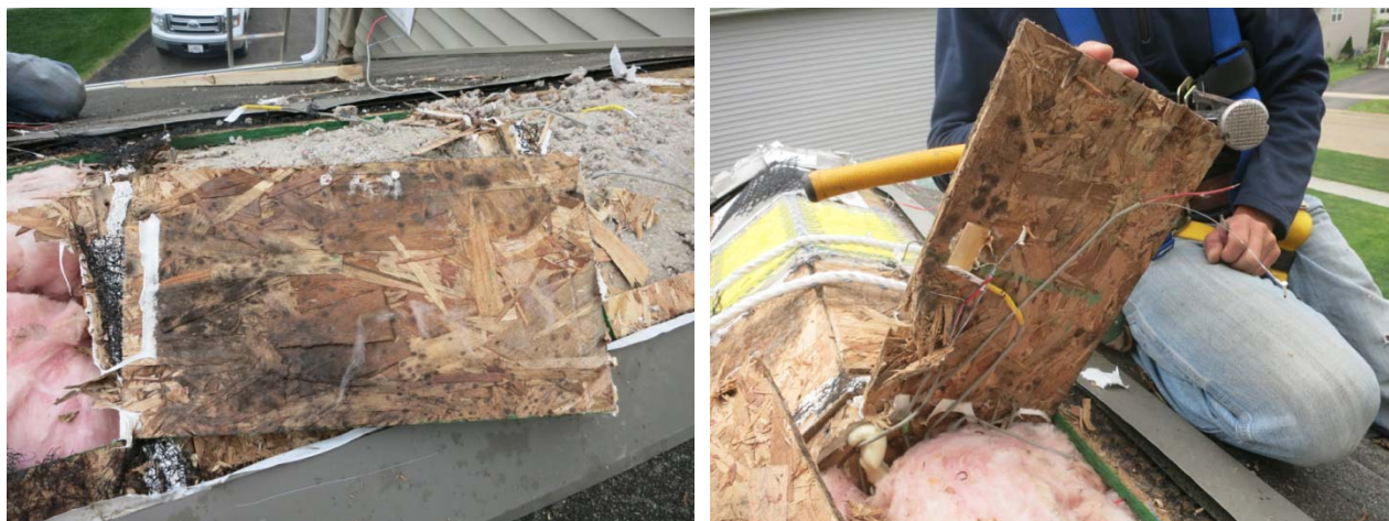
Figure 73: Ridge sheathing bottom conditions, Roof 4
