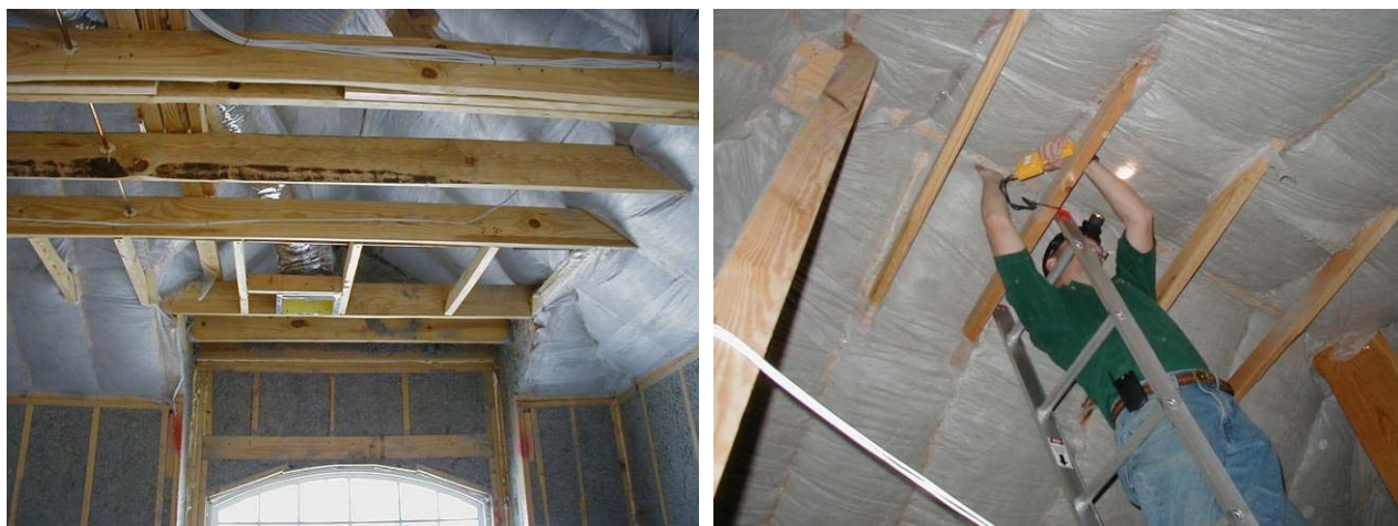
Figure 7: Netted and blown cellulose roof insulation in Houston; moisture content at roof ridge
