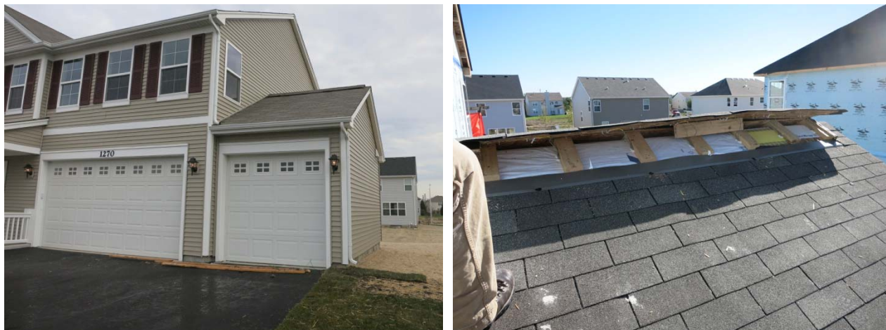
Figure 29: Completed test attic over garage (L), and disassembled “doghouse” detail (R)
