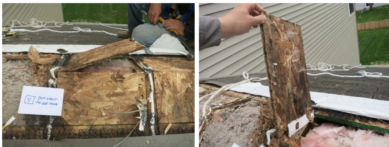
Figure 72: Ridge sheathing top (L) and bottom (R) conditions, Roof 4
