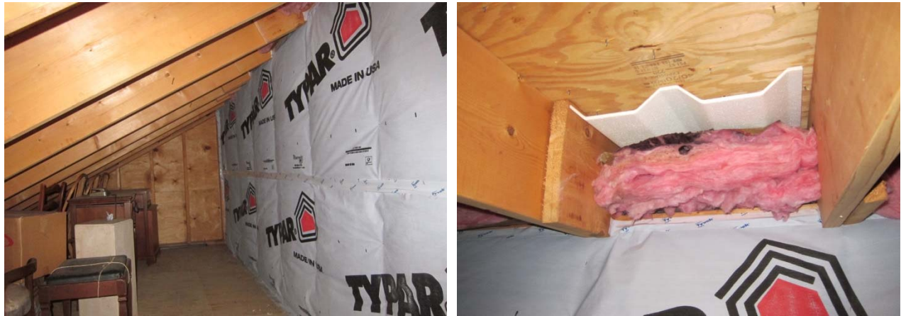
Figure 141: Story and a half compact roof example (with insulation and ventilation chute)
