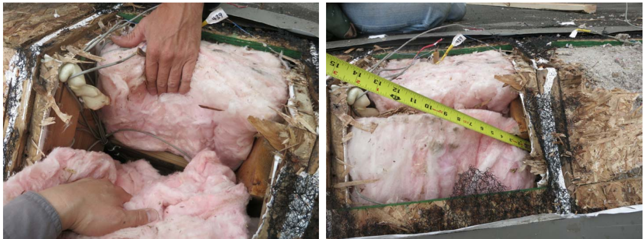
Figure 75: Fiberglass batt conditions at ridge, Roof 4
