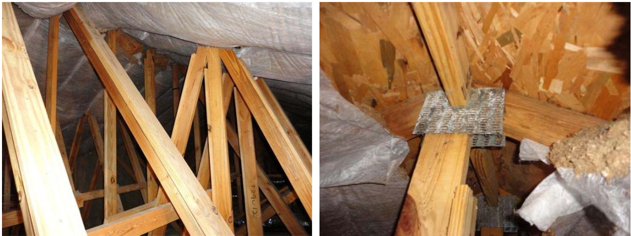
Figure 8: Netted and blown cellulose roof insulation in Jacksonville; corrosion of ridge truss plate
