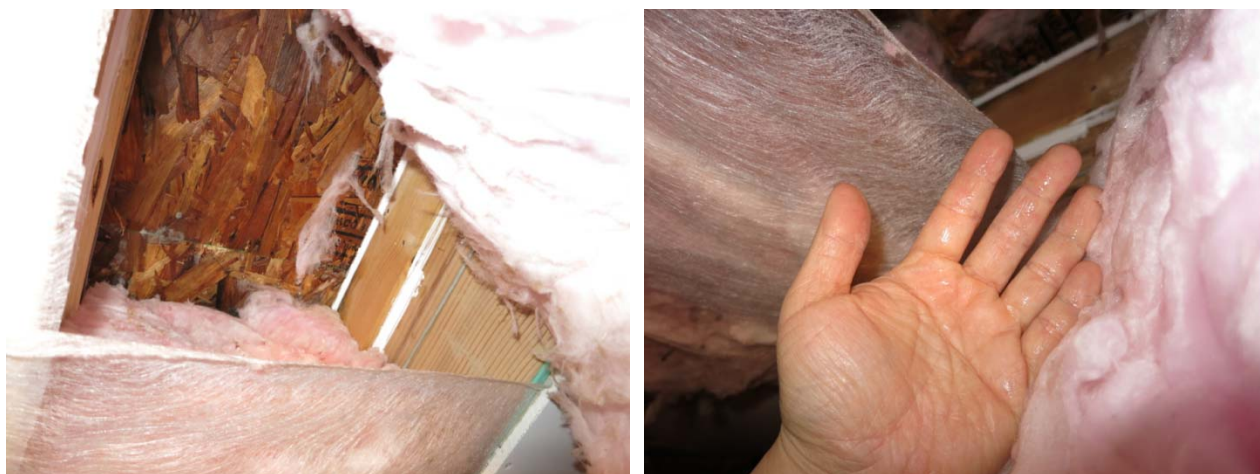
Figure 54: Top vent fiberglass, no GWB (4) wet sheathing (L) and wet batt (R)
