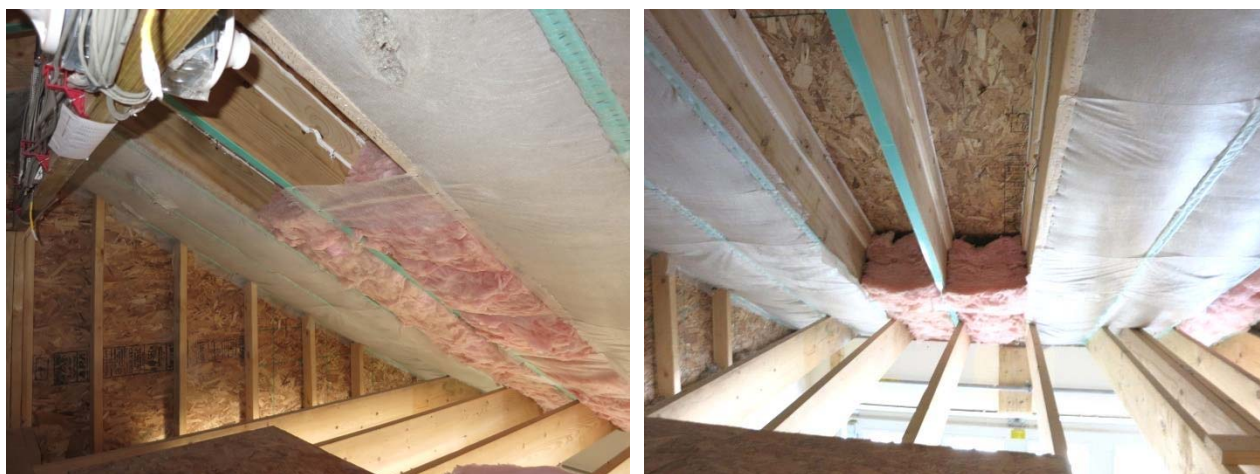
Figure 21: Top vent fiberglass roofs (roofs 4 and 5)
