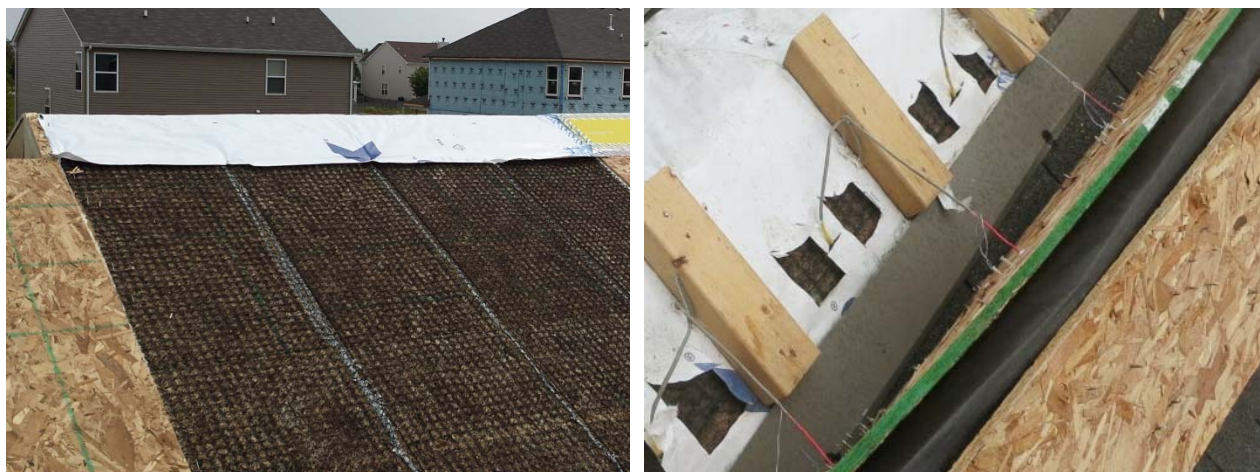
Figure 19: Top vent roof (2, 3, 4, 5) ridge housewrap covering and cut openings
