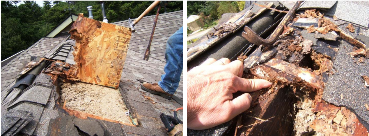
Figure 9: Ridge sheathing degradation with dense pack cellulose in northern California
