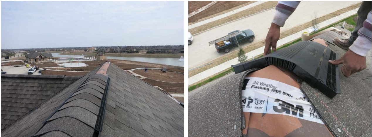
Figure 98: Venting detail at ridge (L) and hip (R), showing vent profile
