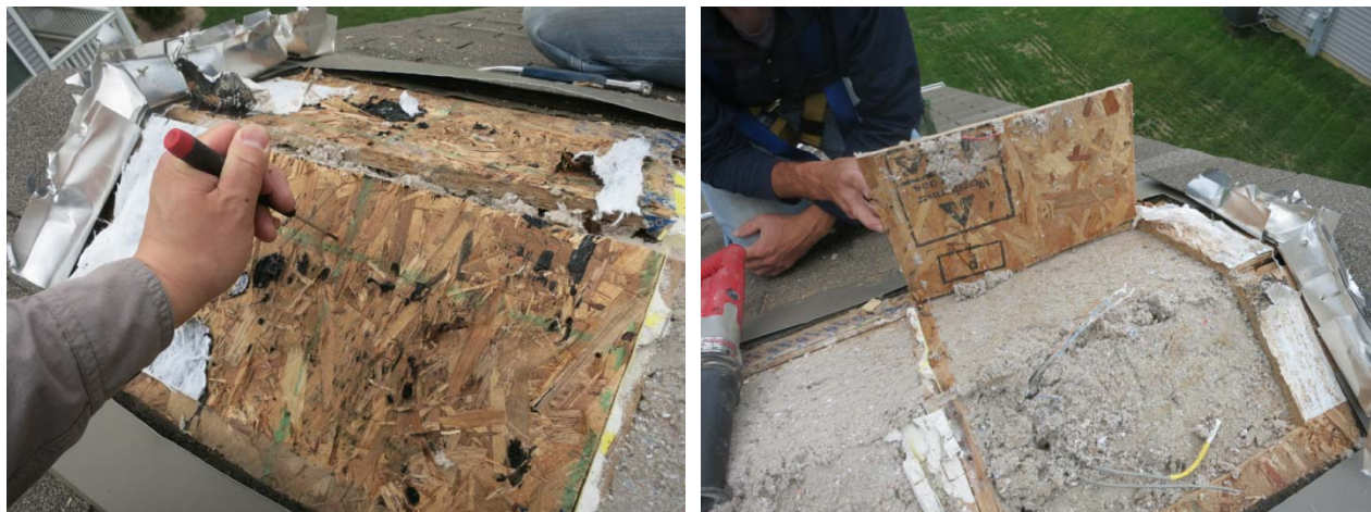
Figure 78: Ridge sheathing top and bottom; cellulose conditions, Roof 7
