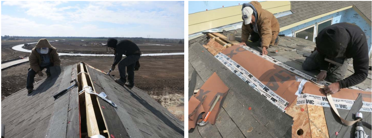
Figure 96: Open ridge (“diffusion port”) detail (L); permeable membrane applied over ridge (R)
