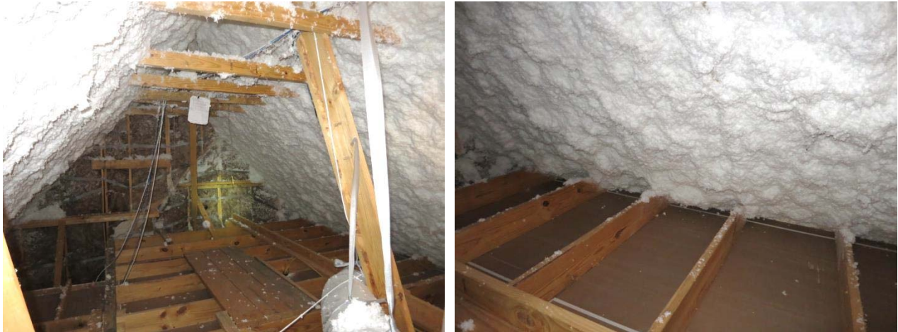
Figure 92: Interior of spray-applied fiberglass insulation in conditioned attic
