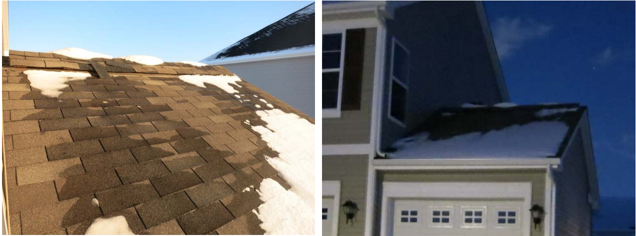
Figure 156: Snow deposits and melting at front (west) orientation of test roof
