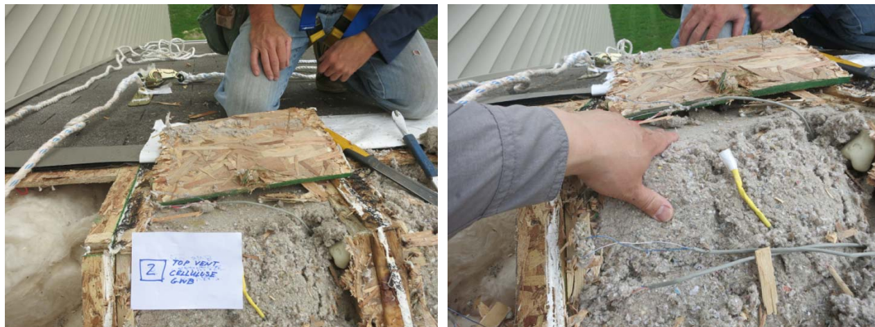
Figure 71: Ridge sheathing top conditions, Roof 2 (L); cellulose conditions (R)
