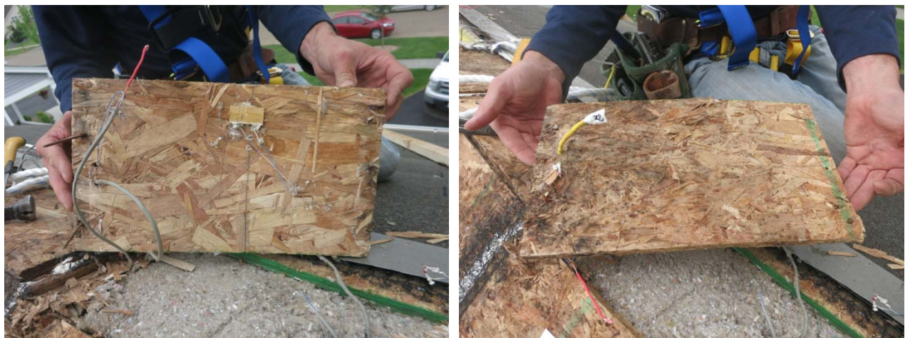
Figure 70: Ridge sheathing bottom (L) and top (R) conditions, Roof 3
