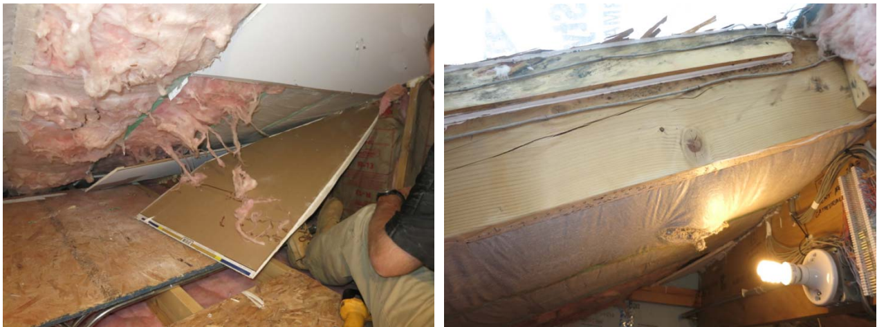
Figure 83: Staining of ceiling gypsum board at (L); mold on framing (R), Roof 5
