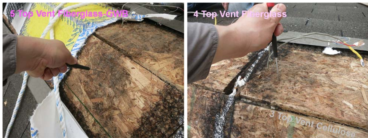
Figure 68: Ridge sheathing conditions (“screwdriver test”) for Roofs 4 and 5
