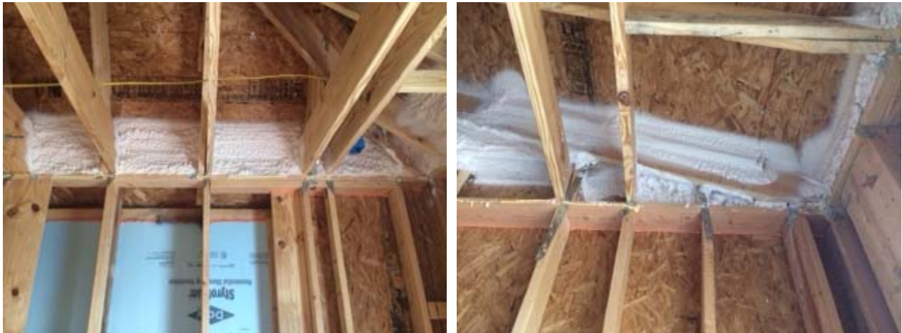
Figure 93: Spray foam used for roof-to-wall air barrier connection
