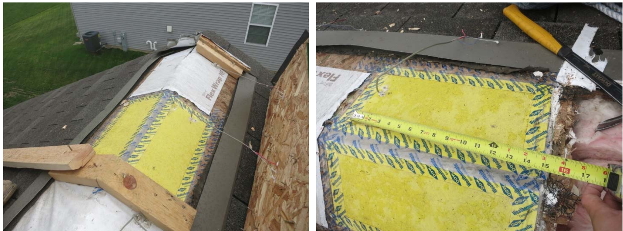
Figure 24: Diffusion vent (6) and unvented (7) ridge conditions
