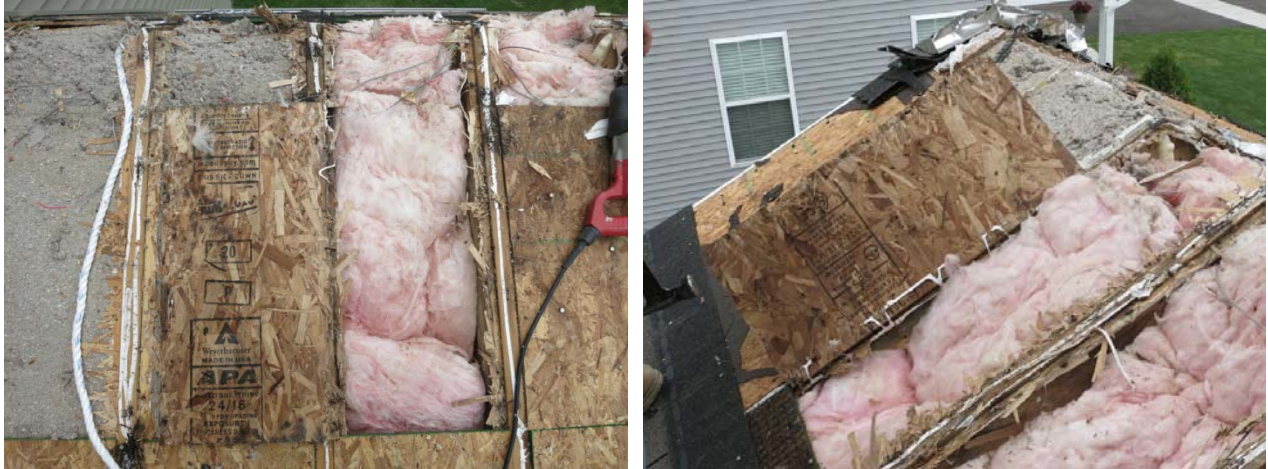
Figure 82: Sheathing away from ridge, Roofs 4 (left) and 5 (right)
