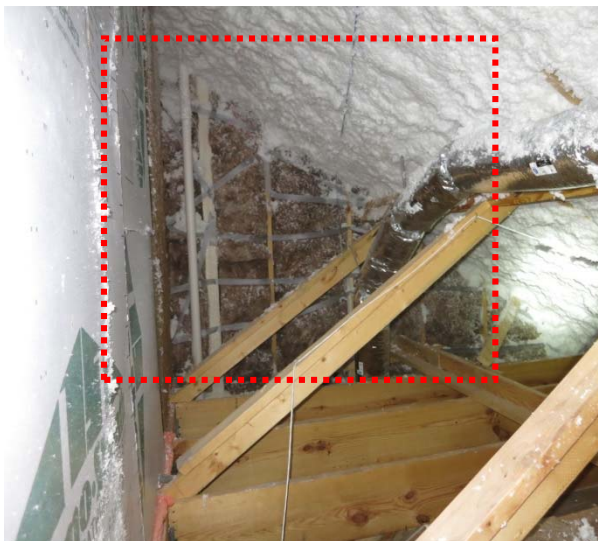
Figure 112: Air leakage at rear attic over master bedroom (Location D)
