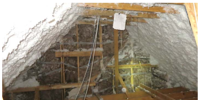
Figure 109: Air leakage at front attic gable end (Location B)
