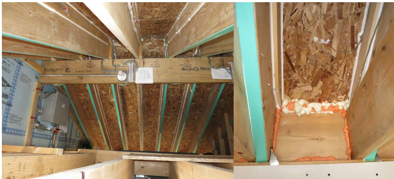
Figure 30: Interior of experimental roof bays, showing air sealing, gaskets, and instrumentation
