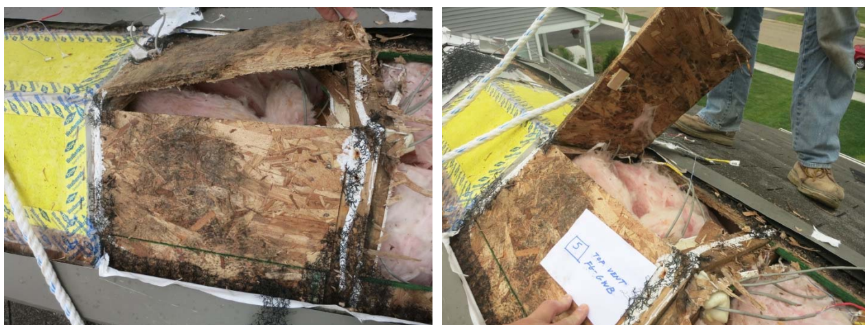
Figure 74: Ridge sheathing conditions, Roof 5
