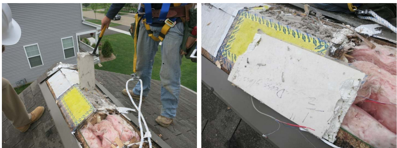
Figure 77: Ridge sheathing top and bottom conditions, Roof 6
