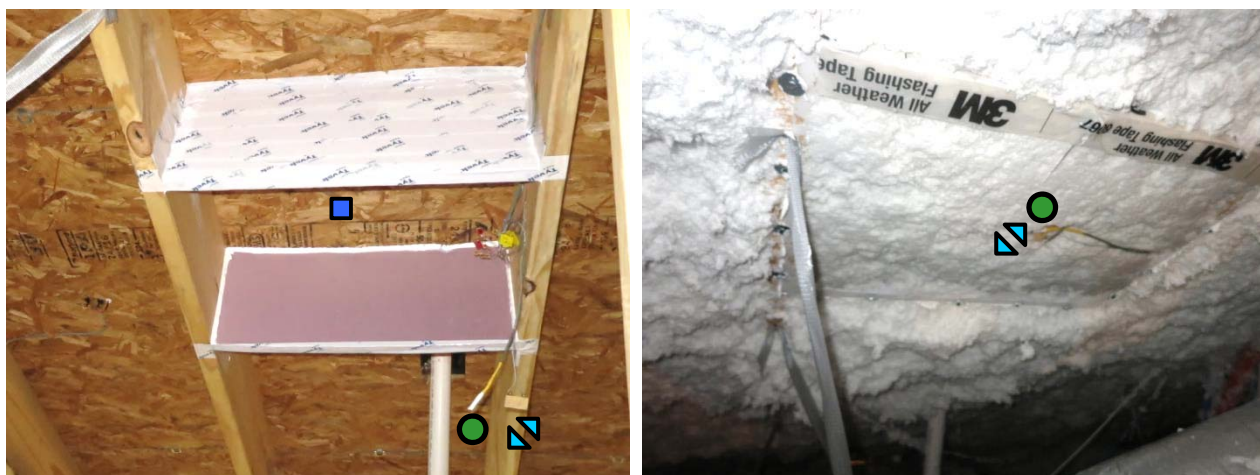
Figure 104: Inward drive “box” before insulation (L); after insulation and clear plastic cover (R)
