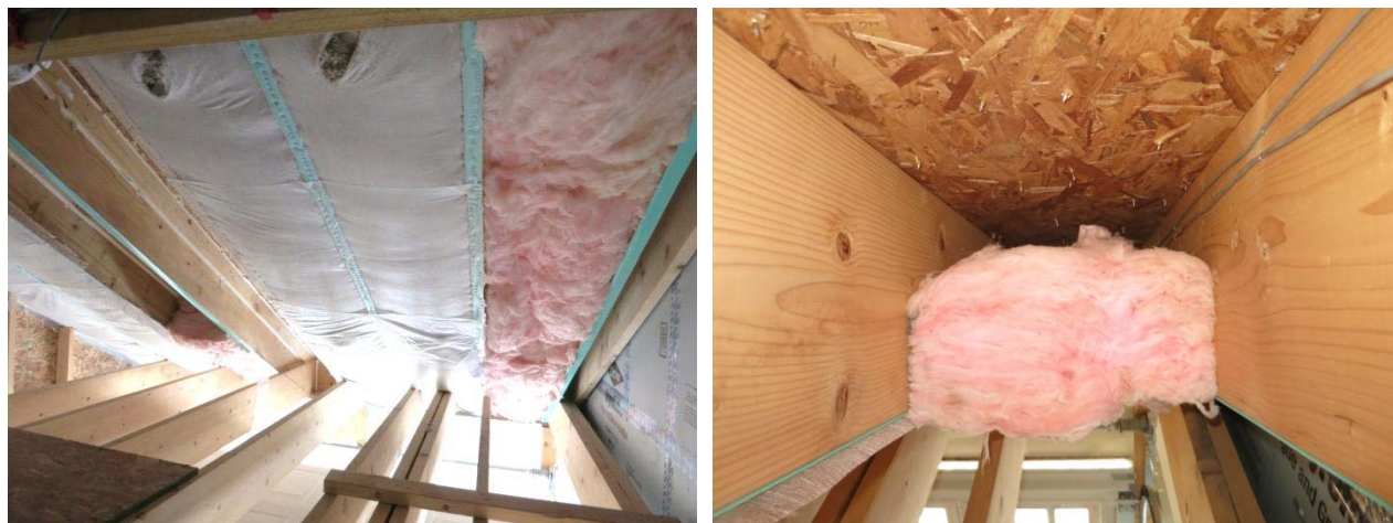
Figure 15: Roof 1-Vented compact roof insulation, showing airspace/ventilation detail
