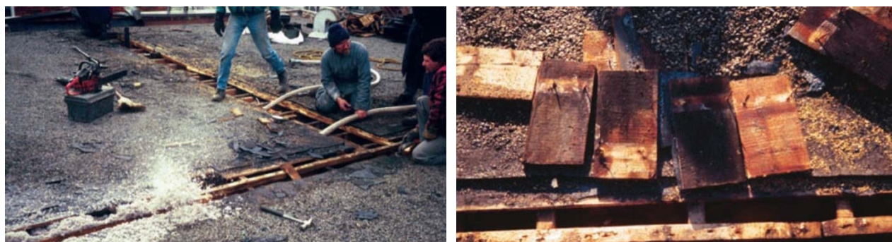
Figure 1: Dense pack insulation of roof (L) and resulting moisture issues (R) Lstiburek (2010b)
