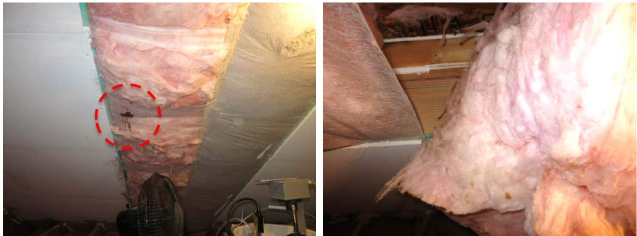
Figure 53: Top vent fiberglass, no GWB (4) water leak (L) and wet fiberglass batt (R)
