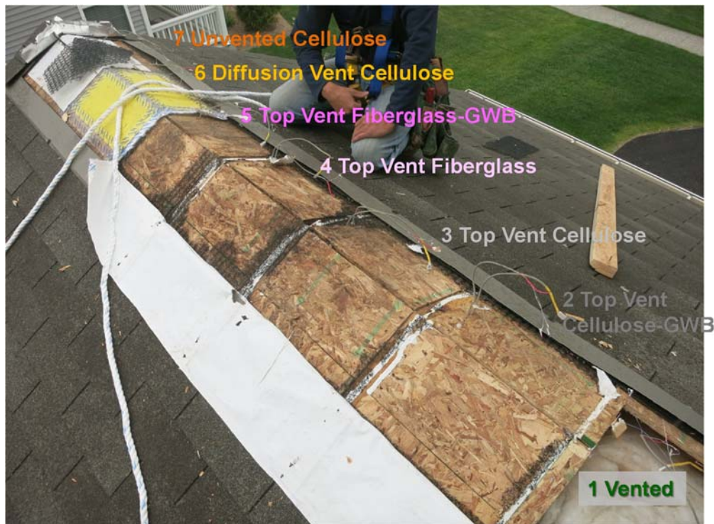
Figure 67: Ridge conditions, after removal of breather mesh
