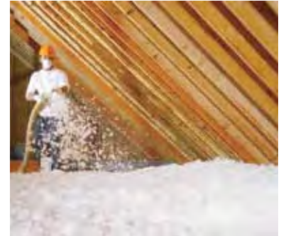
In attic applications, EcoFill Wx blows smooth and fast, providing superior coverage.
