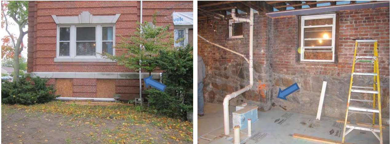
Figure 12: BSMT-W1 and BSMT-W2 joists, showing water deposition at wall jog
