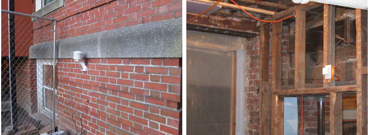
Figure 24: Exterior (left) and interior hallway (right) temperature/relative humidity sensors
