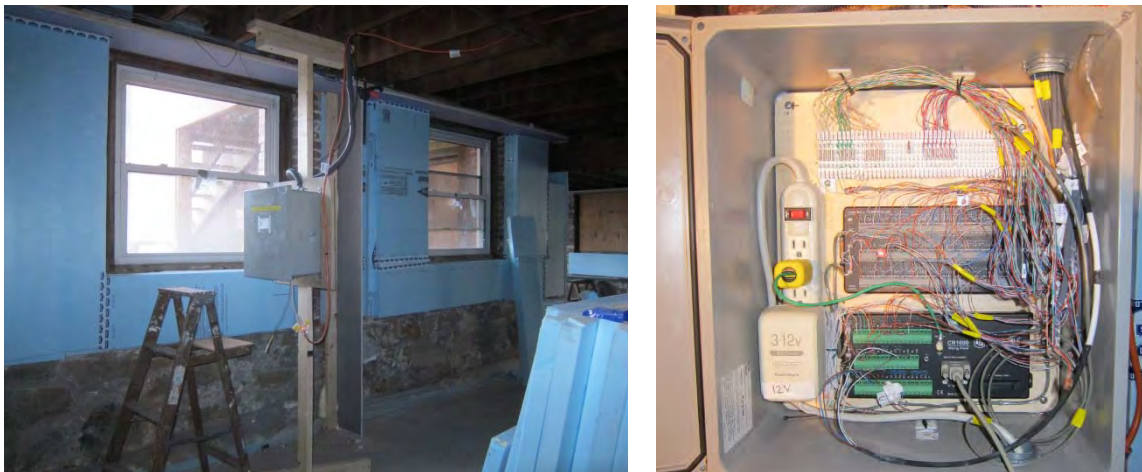
Figure 25: Data acquisition system, showing placement (left) and wiring connections (right)
