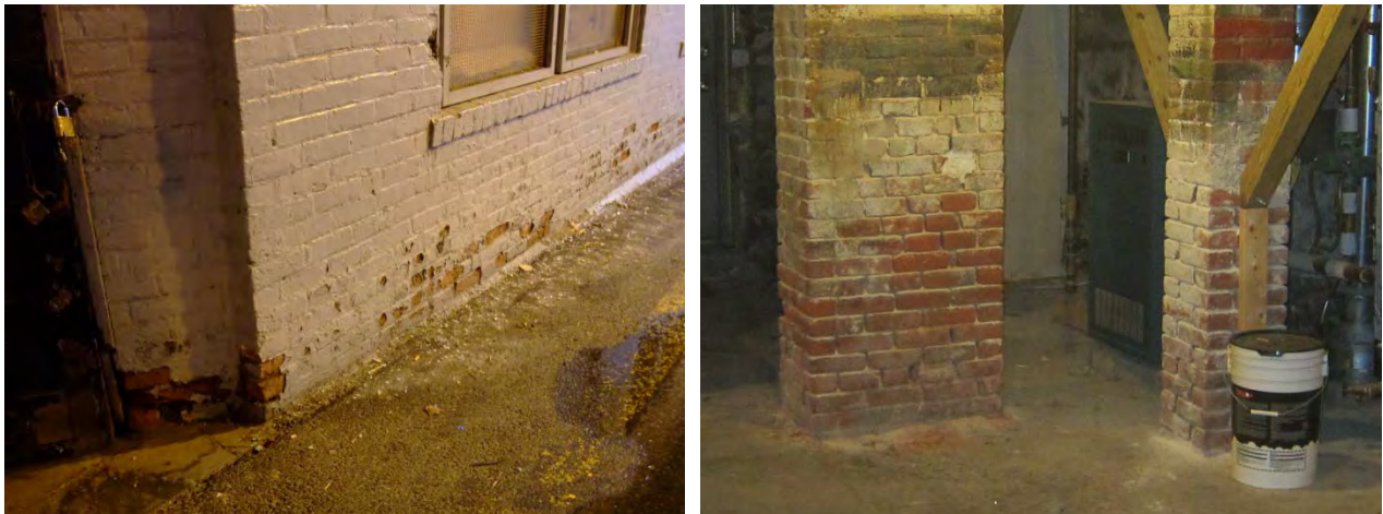
Figure 55: Suspected de-icer salt damage (left) and basement capillary rise damage (right)
