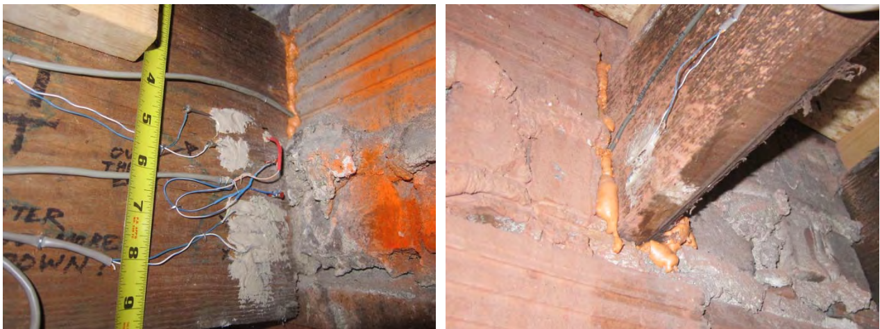
Figure 21: Caulked pocket holes (left) and air seal at joist pocket (right)
