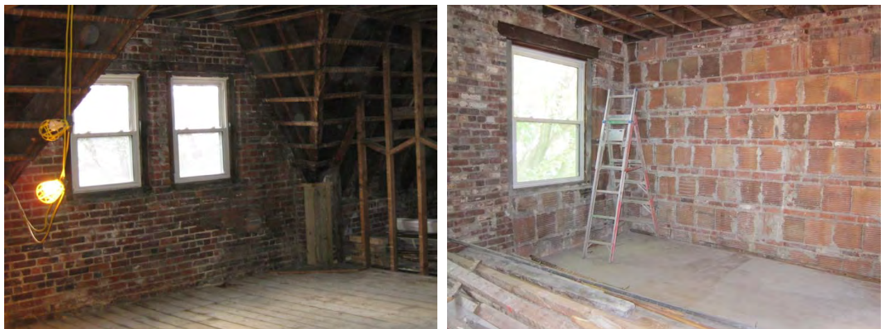
Figure 4: Exterior wall conditions at solid brick (left) and hollow clay block infill (right) conditions
