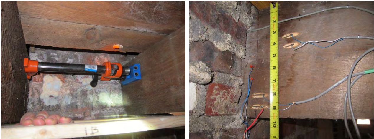
Figure 20: Pocket hole jig (left) and installed moisture content pins (right)
