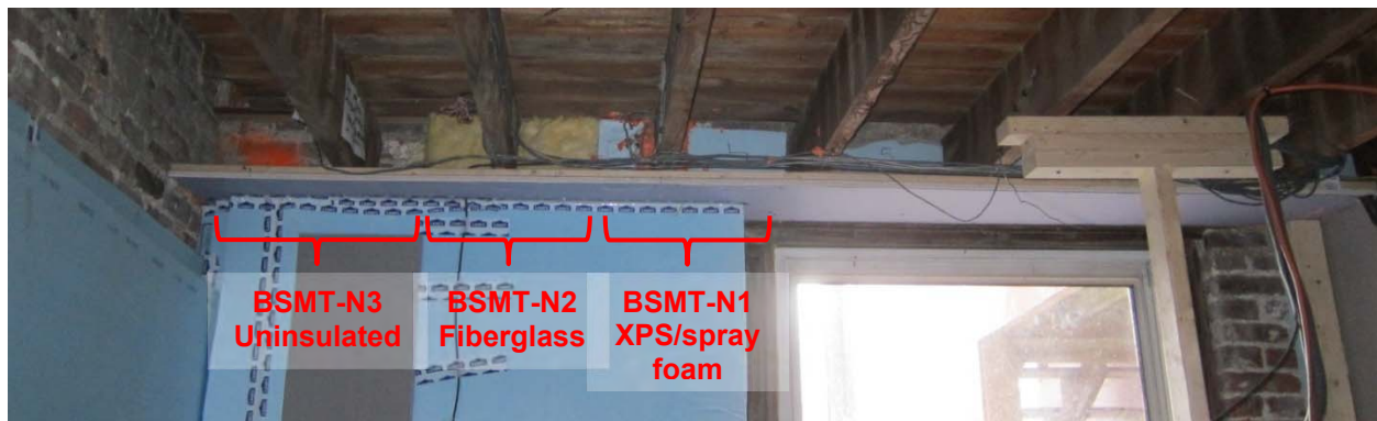
Figure 9: Comparison of insulation strategies for joist ends BSMT-N-1/2/3, pre-drywall
