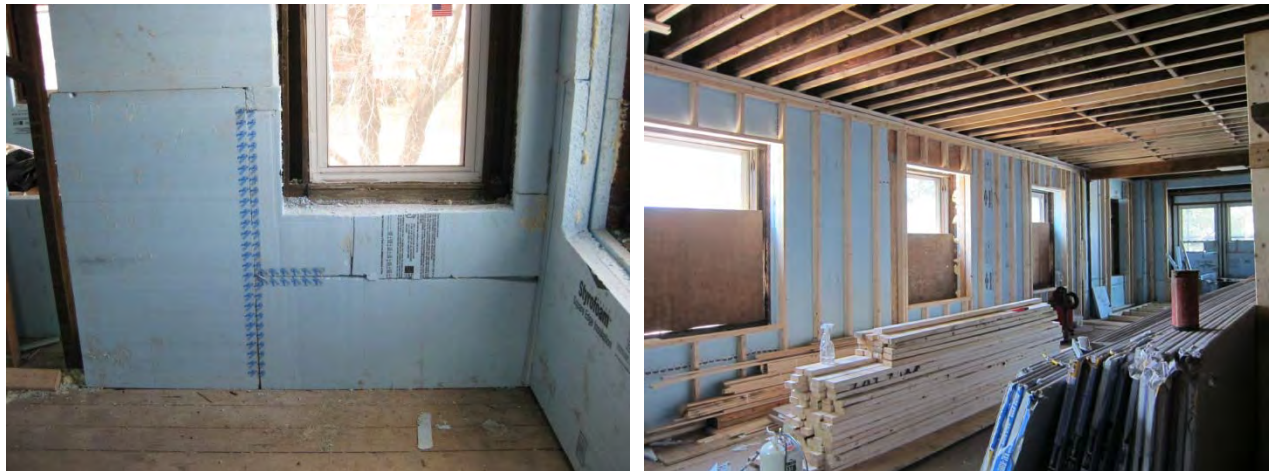
Figure 6: Multiple layers of insulation (left) and framing installed inboard of insulation (right)
