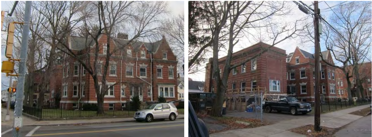
Figure 1: Merrimack Valley Habitat for Humanity retrofit building from west (left) and north (right)
