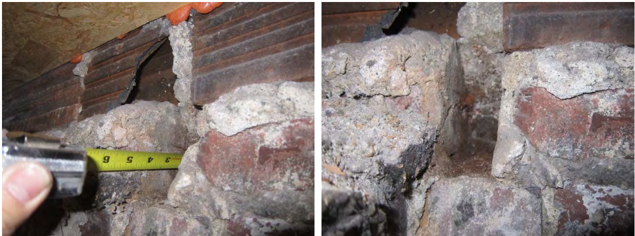
Figure 23: Conditions in joist pocket at north-facing building at addition
