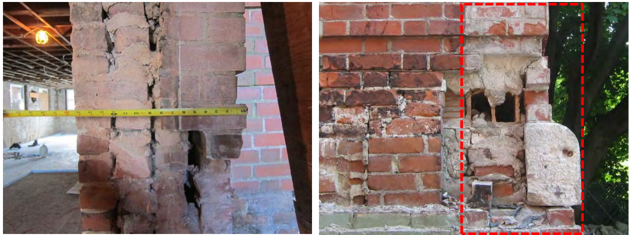
Figure 5: Wall section at solid brick (left) and at hollow clay block infill (right) conditions
