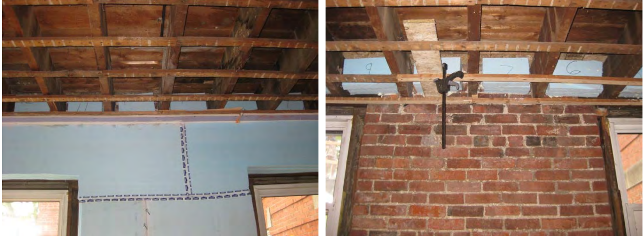
Figure 7: Embedded joist foam blocks (left); close-up showing clamping jig (right)
