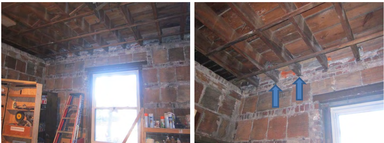
Figure 13: FIRST-N joists, showing brick and clay block wall construction
