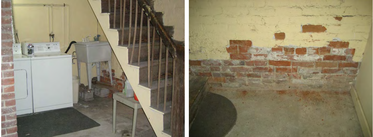
Figure 56: Brick spalling and paint blow-off basement party wall due to capillary rise
