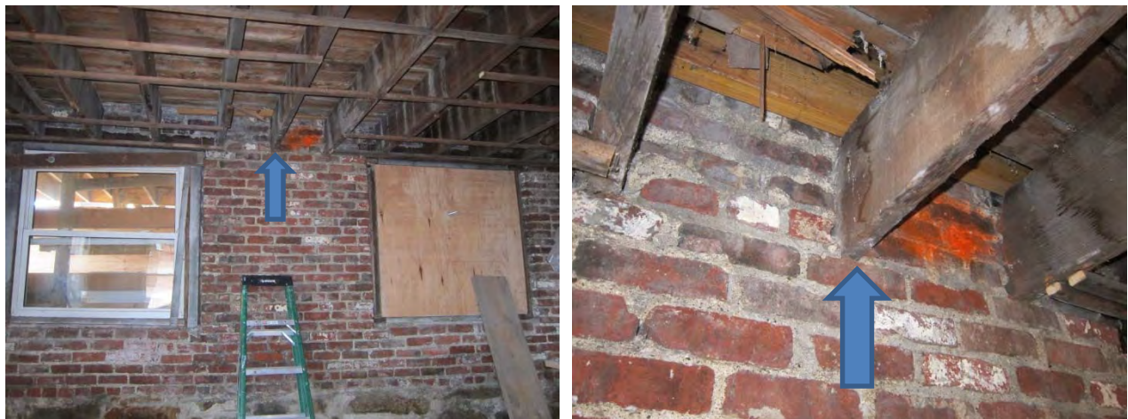
Figure 11: BSMT-E-2 joist, showing existing water staining
