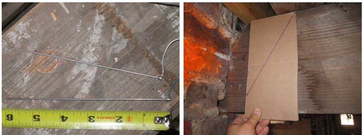
Figure 19: 6” extended moisture content pins (left) and determining drilling depth (right)
