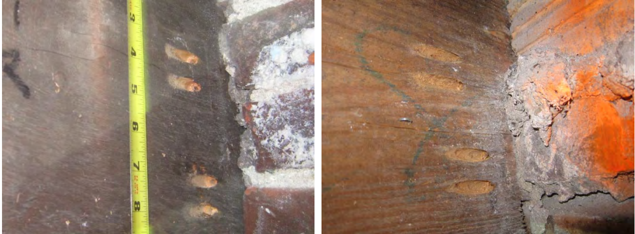
Figure 14: Wood color comparison at BSMT-E-1 and FIRST-E joists
