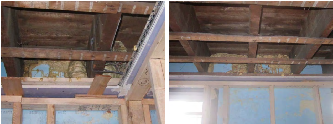
Figure 15: Two-component spray foam air seal at joists BSMT-W1 and BSMT-E1
