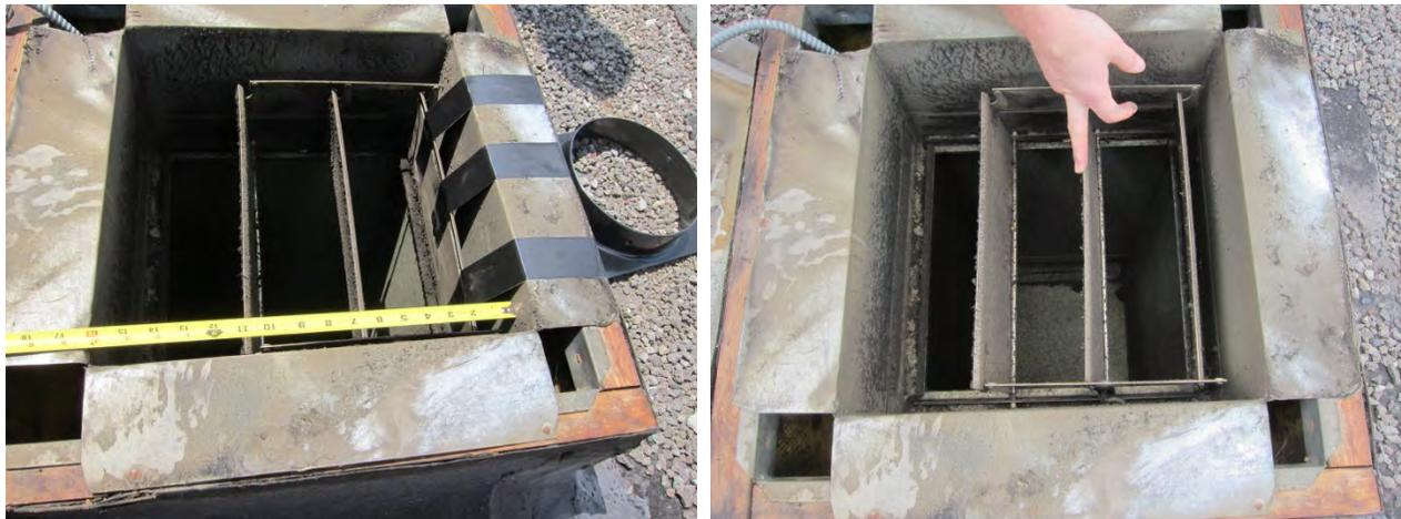
**Figure 31. Spring-loaded louvers on exhaust fan rooftop curb blocked open at EF-1 testing**
