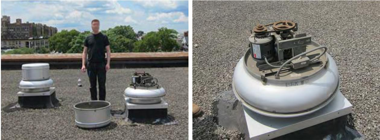
Figure 27. Typical rooftop exhaust units (L); cover removed from exhaust fan (R)
