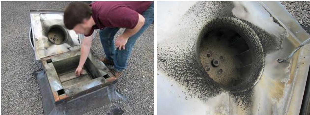
**Figure 29. Open corners at exhaust shaft rooftop curb (L), with dust marking patterns (R)**
