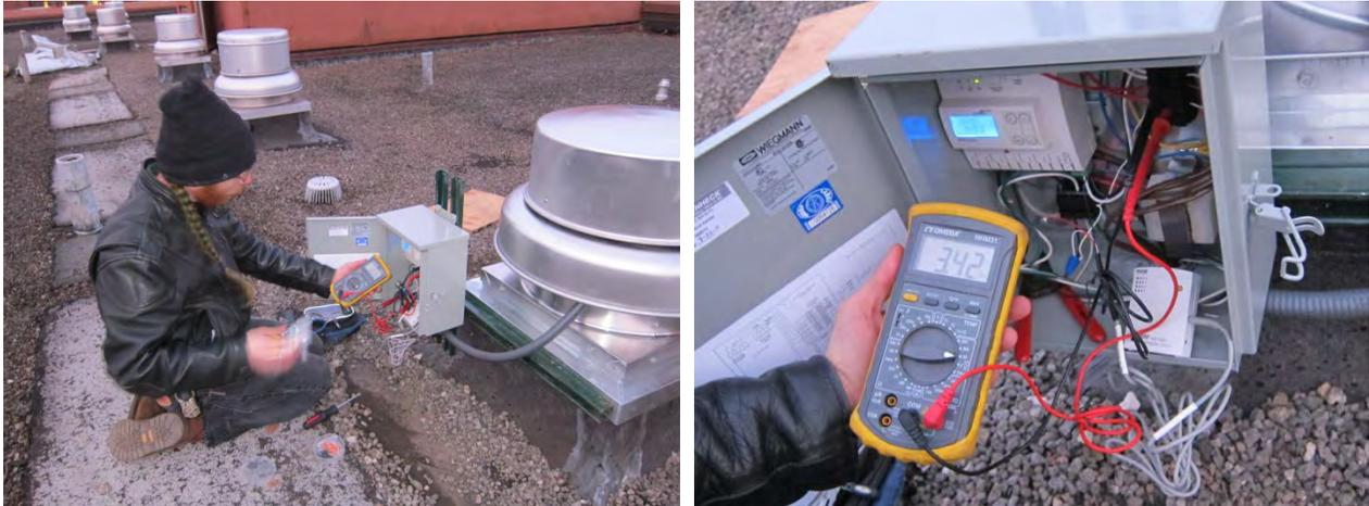
**Figure 77. Installation of voltage data logging equipment on variable speed fans**
