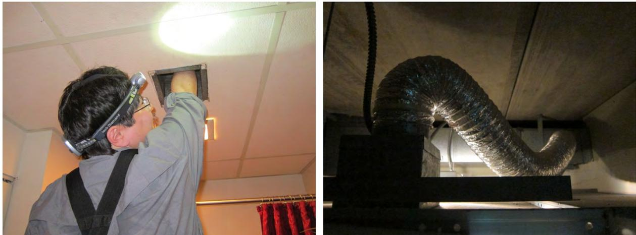
**Figure 17. Typical bathroom register (L) with flexible duct connection to exhaust trunk (R)**
