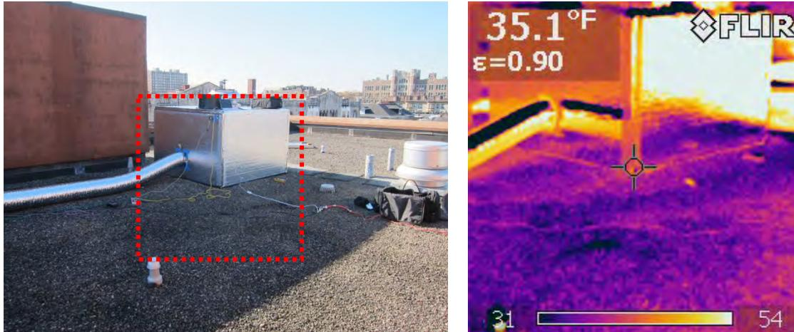
**Figure 55. Powered flow capture hood with infrared, showing minimal leakage at seal**
