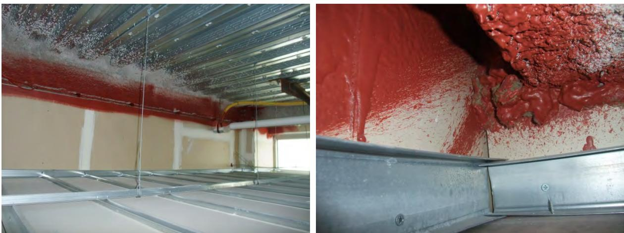
**Figure 49. Liquid spray-applied fire-rated sealant**
