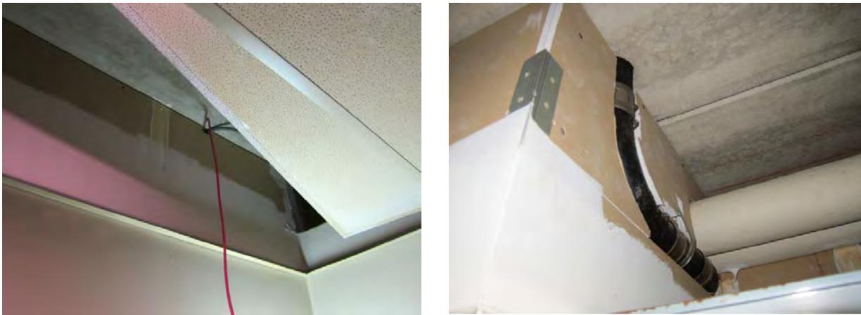
**Figure 47. Lack of air sealing at demising wall to concrete plank (L) and pipe penetration (R)**
