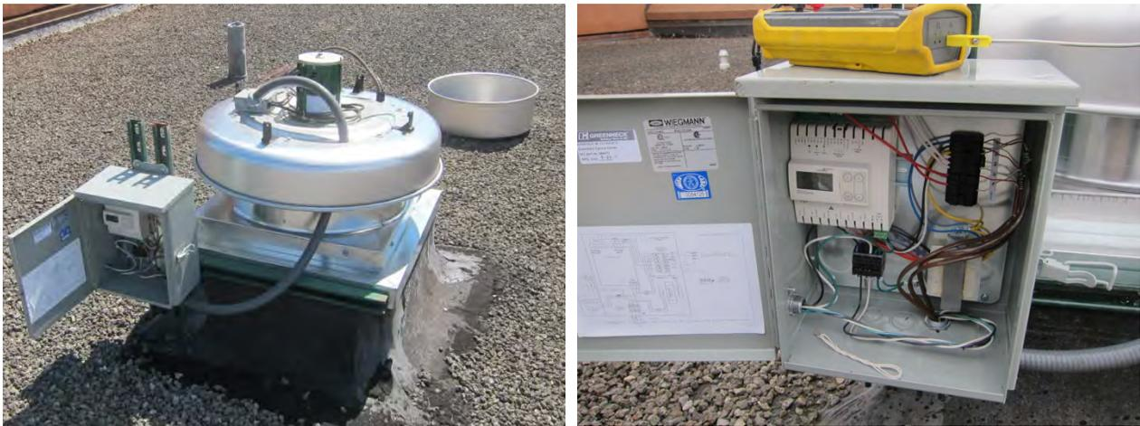
**Figure 50. Variable-speed exhaust fan with cover removed (L), with controller box (R)**
