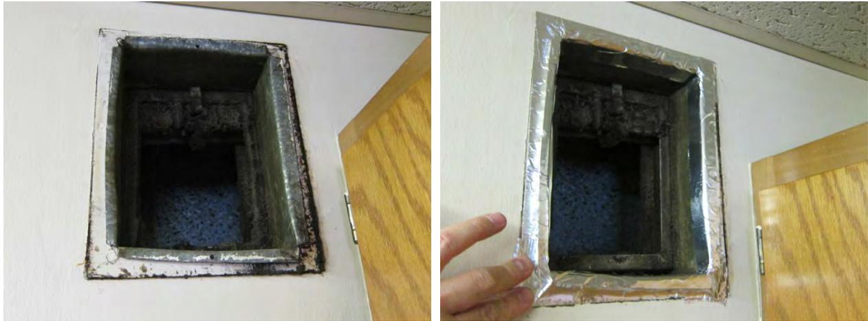
**Figure 30. Kitchen exhaust boot-to-drywall as found (L) and retrofit seal (R) state**
