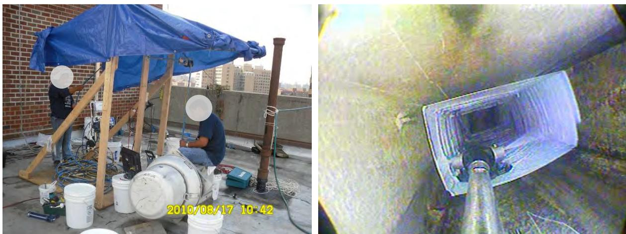
Figure 25. Remote shaft-sealing spray mastic system
