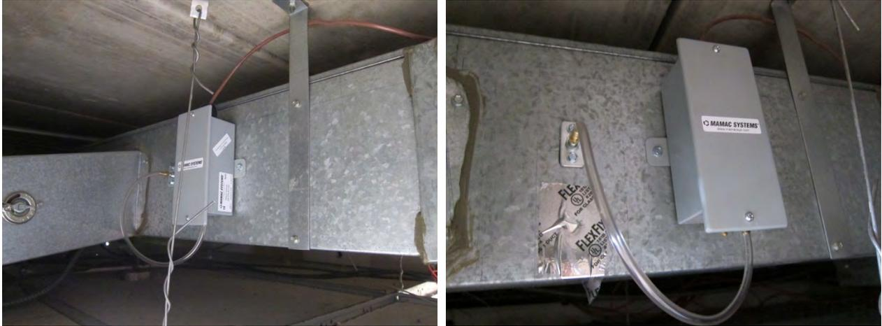
**Figure 51. Duct pressure transducer and static pressure probe on top floor trunk duct**
