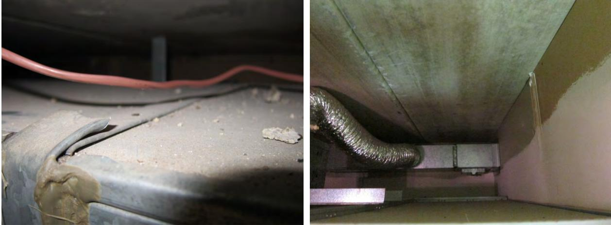
**Figure 33. Limited mastic sealing at sheet metal joints (L); connection to flex runouts (R)**
