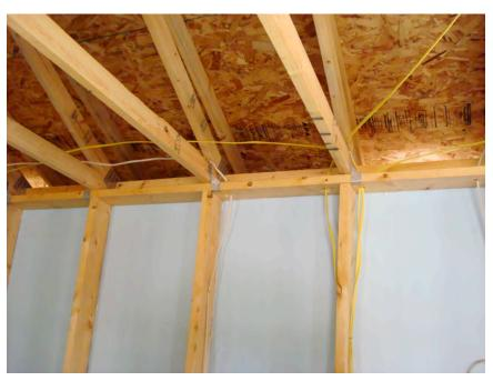
Figure 3.3: Photograph of advanced framing showing single top plate and insulating sheathing
