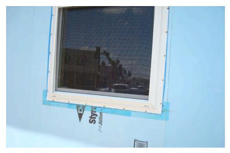
Figure 3.4: Photograph of partially complete window flashing
