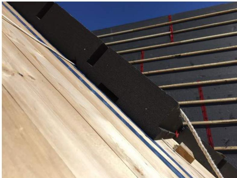
**CLT is Not Airtight - Don't Forget the Membrane**
