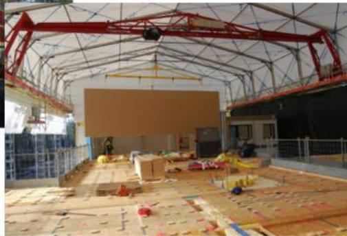
Finland - use of climbing roof and overhead cranes - high degree of modular moisture sensitive components
