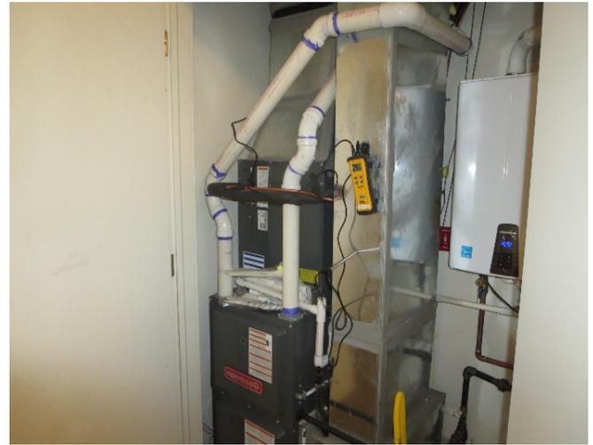
**Figure 23:** Air handler closet in apartment units
