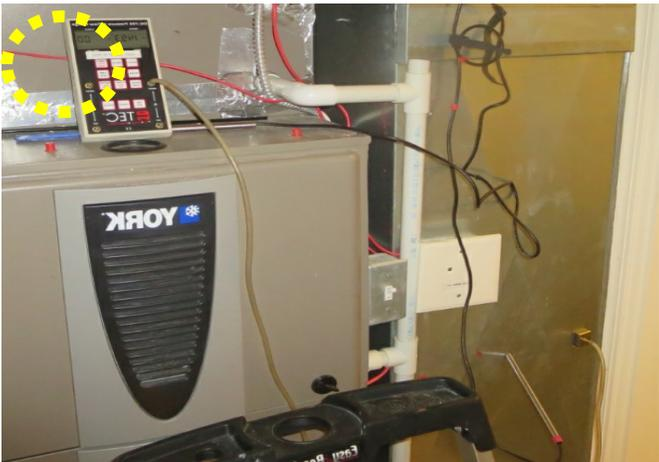
Figure 21: Measuring static pressure
