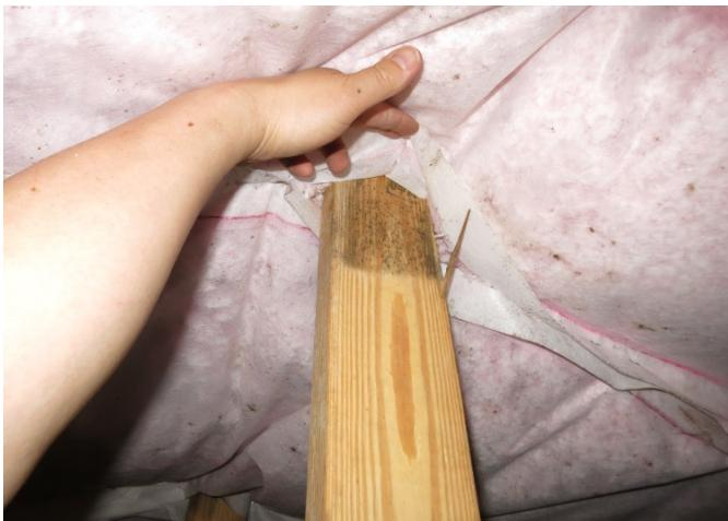
**Figure 9:** Mold on truss top vertical member
