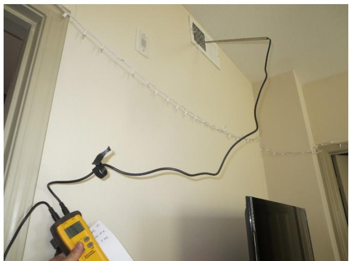
**Figure 14:** Measuring “split” at supply
