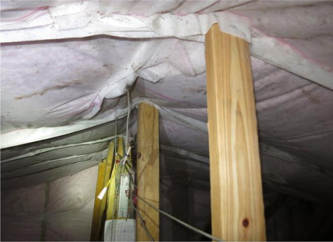
Figure 8: Mold spotting on netting near ridge
