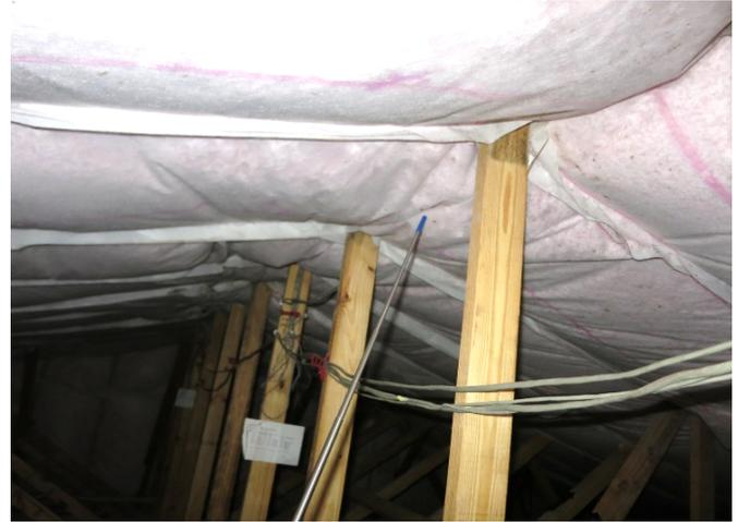
Figure 10: Measuring T and DP stratification
