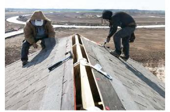
Photograph 8: Vent Opening In Roof Sheathing— Standard construction practice is used to provide vent opening at ridge area.
