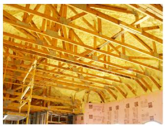
**Photograph 1: Spray Polyurethane Foam**—The typical technology to make the inside bigger is to construct conditioned attics using spray polyurethane foam. We have been using low-density and high density SPF in this way for over 20 years with good success.
