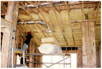
**Photograph 11: Fiberglass Batts** – Works with fiberglass batts.
