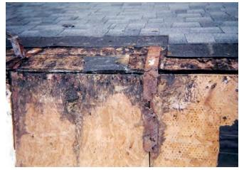
**Photograph 3: Classic Ridge Rot** – If you "caught it" in the first couple of years before it spread you could save the roof with a vapor diffusion vent.
