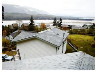
**Photograph 2: Juneau, Alaska** – SIP roof assemblies in a cold climate where annual rainfall is measured in feet not inches.
