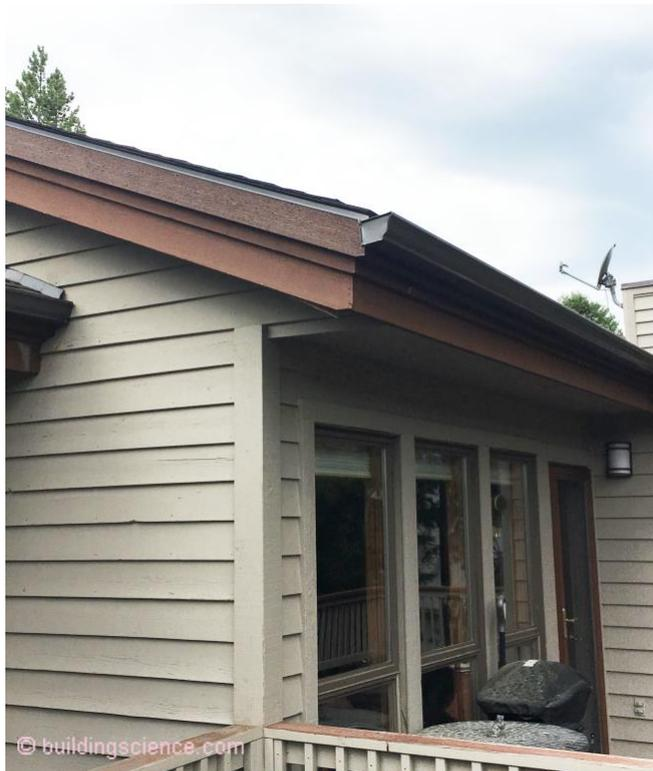
**Photograph 7: Vented Over Roof Soffit** - The fascia detail is continuous and unobtrusive.
