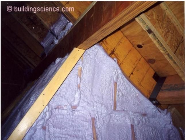
**Photograph 5: Skylight Shaft** - If you have sky lights you have to air seal and insulate the shafts big time. In a retrofit situation I know of no easier way than going the SPF route.
