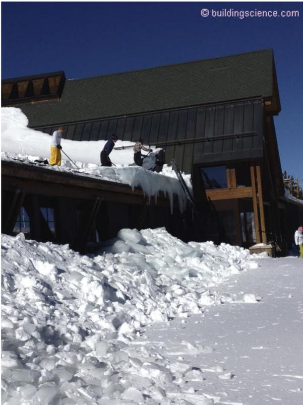
**Photograph 10: Hacking Away at Ice Dams -** Big time damage to your roof when you hack away at the ice dam.
