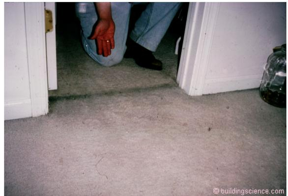
**Photograph 1: Carpet as a Filter** - Discoloration of carpeting due to particulate accumulation.
