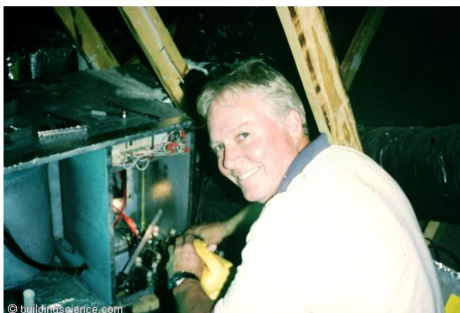
**Photograph 7: Smiling Guy** - Chuk Bowles cleaning the key surfaces in an air handling unit 30 years ago. Good to be correct, eh?
