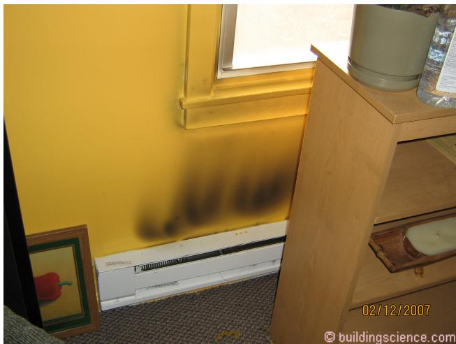
**Photograph 6: Electric Resistance Baseboard Heaters** – What a mess... an energy efficient respirable particle generator.
