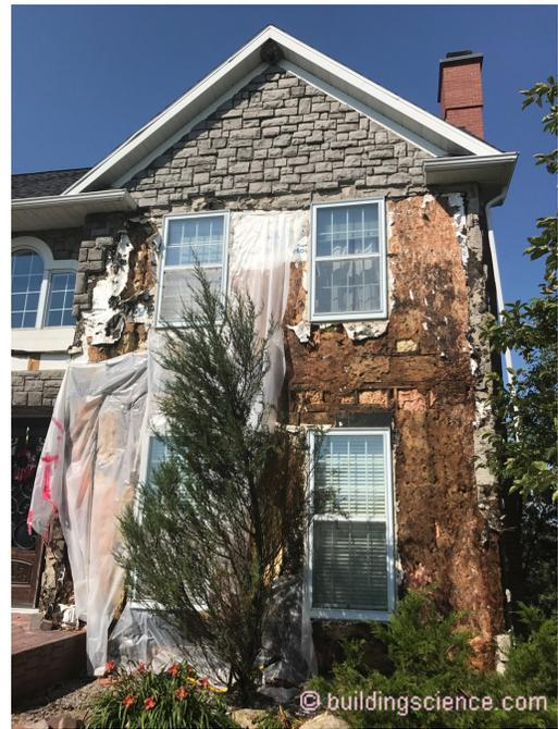
**Photograph 1 – Lumpy Stucco Disaster:** Stucco layer with adhered stone installed over a synthetic building paper over oriented strand board sheathing (OSB). Water held in nooks and crannies leads to a greater water load than traditional stucco. No drainage or capillary break or hygric redistribution.
