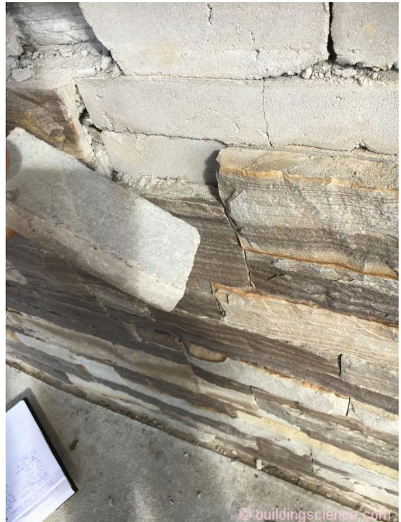
**Photograph 5 – Thin Stone Veneer Adhesion Failure:** Bond failure is at the veneer-thin set interface.
