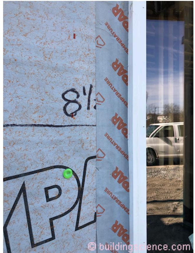
**Photograph 5: “Bumpy” Housewraps** - The “bumps” create a drainage gap that provide a drainage efficiency of greater than 90 percent, as measured in accordance with ASTM E2273 or Annex A2 of ASTM E2925. The “bumps” also provide for lateral and vertical hygric redistribution.
