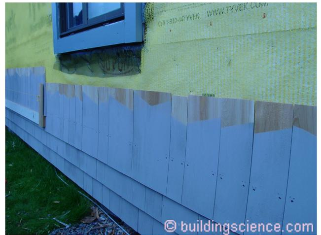
**Photograph 1: Thousands of Holes** - Cedar shingles nailed through a housewrap water control layer resulting in thousands of holes on a large house on the ocean in New England. But the wall assembly does not leak because the hydrostatic pressure driving force is controlled by the drainage mat installed between the cedar shingles and the mechanically attached water control layer....resulting in....wait for it...”drainage”.
