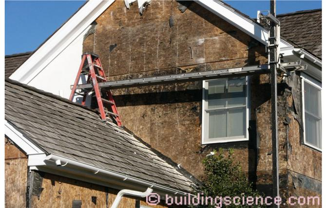
**Photograph 2: Stucco Failure** – Not a pretty sight. No drainage coupled with moisture sensitive sheathing (oriented strand board – OSB) and high levels of thermal resistance (not enough energy flow to facilitate drying).
