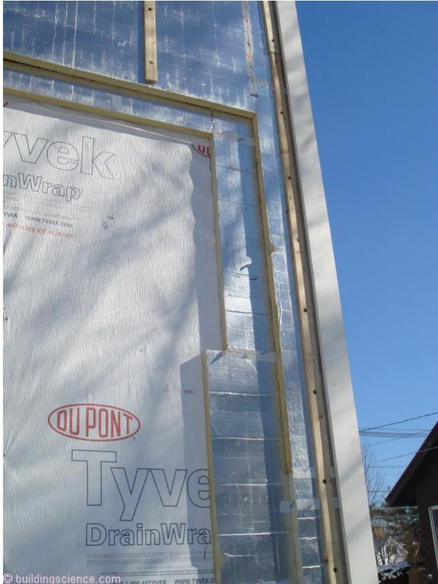
**Photograph 1: Gap Behind Continuous Exterior Insulation** - There are “draining housewraps” and “draining wrb’s”... basically “textured” sheet goods that create a space or a gap.
