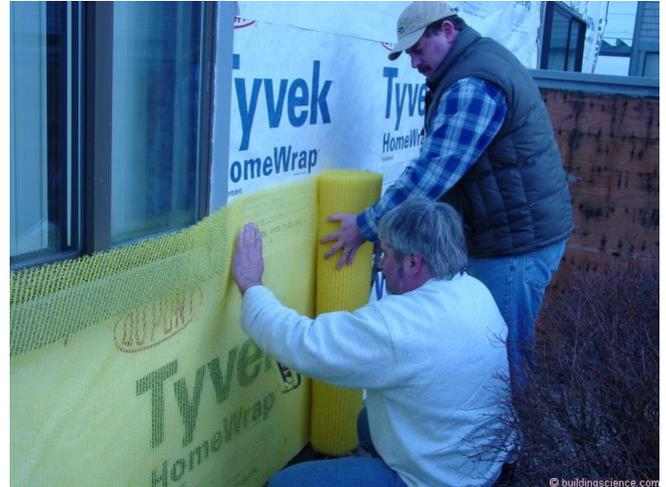
**Photograph 4: Drainage Matt for Wood Shingle Cladding** – Wood shingles need a drainage gap of at least 3/16 inch. Most drainage mats are ¼ inch to 3/8 inch so they work well.
