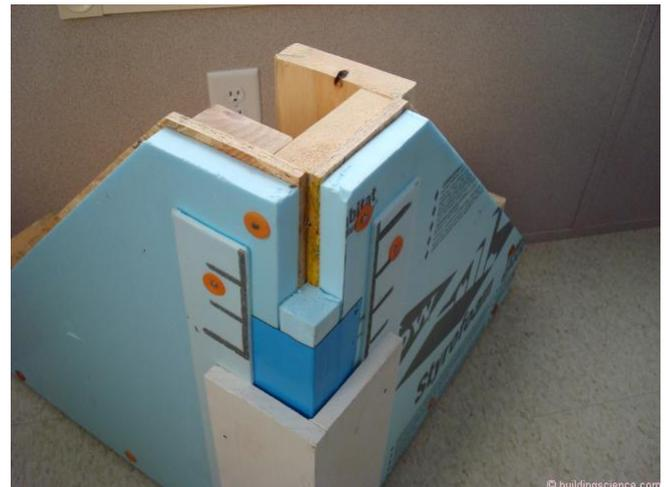
**Photograph 5: Furring for Fiber cement or Wood Based Siding** – Fiber cement or wood based siding need a drainage gap of at least 3/16 of an inch.
