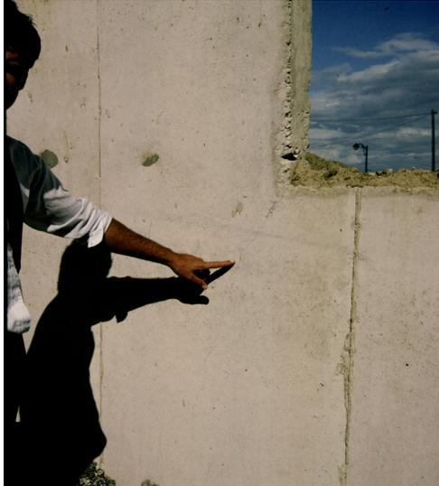
**Photograph 3: Concrete Crack** – Cracking typically happens at stress concentrations such as at punched openings. The hand pointing to the crack belongs to a young (at the time) James Lischkoff...before he became a famous Canadian building scientist.
