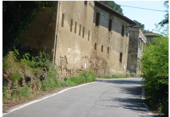
**Photograph 2: Abandoned Buildings** - Surprisingly many buildings are abandoned and in disrepair. Spalling of renderings is typical. Rainwater management is poor. Flashings are non-existent.
