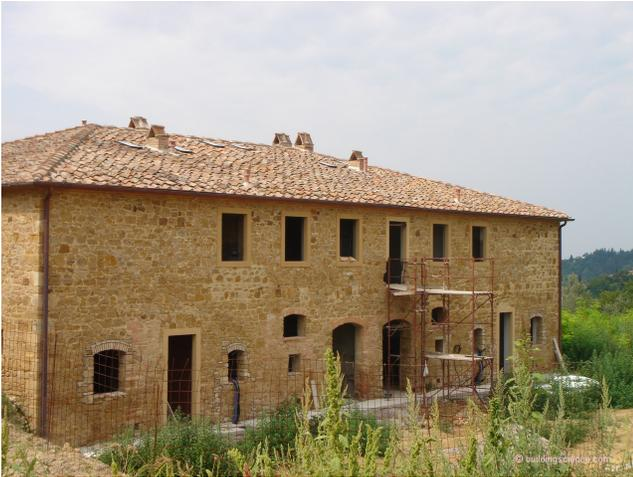
**Photograph 7: Tuscan Roofs** – Tile roofing. Notice the rain shedding chimney caps.
