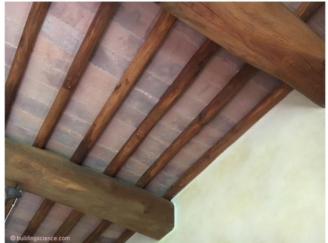
**Photograph 6: Tuscan Roofs** - Terracotta bricks supported by wood rafters and wood timber beams.
