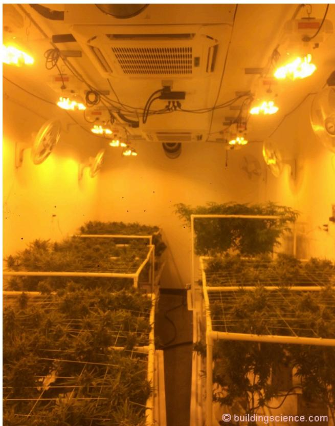
**Photograph 4: Commercial Grow Operation** – Humidified, pressurized, temperature controlled, carbon dioxide injected, lighted, circulated...easy right?
