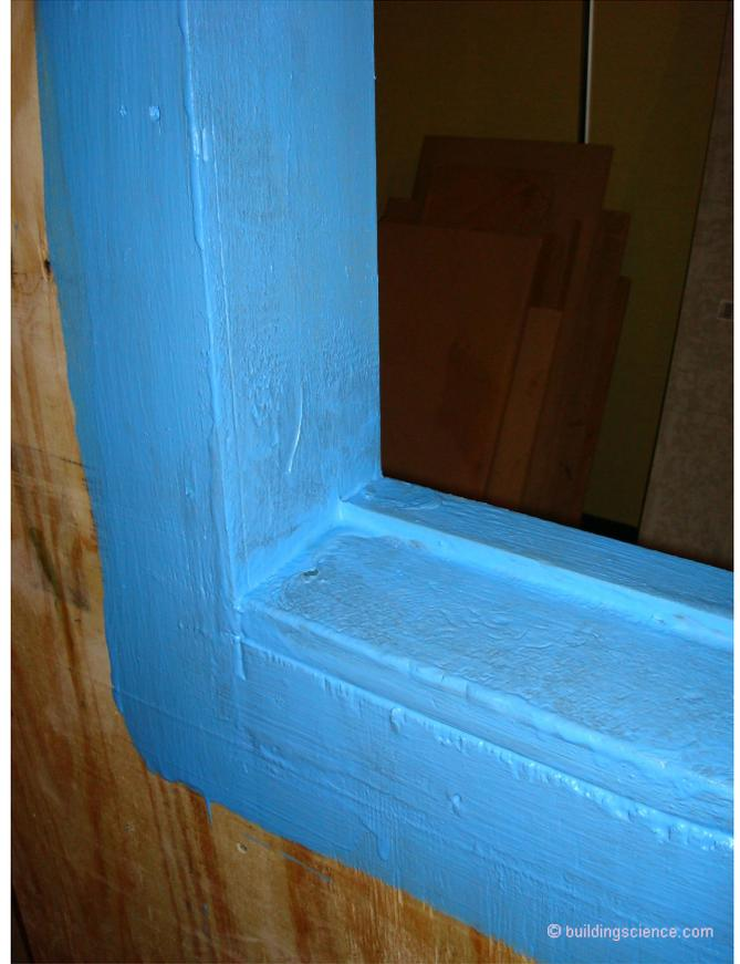
**Photograph 4: Window Opening** – Lots of joints and inside and outside corners. How we deal with the joints and the inside and outside corners is the trick. Note the “file” sealant in the “end dam” and “back dam” under the liquid applied membrane.
