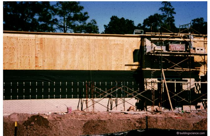
**Photograph 5: Old School** - Apparently a point missed by folks is that we installed asphalt impregnated felt, Type D coated building papers and building wraps by nailing and stapling them and then we nailed and screwed cladding systems through them and did nothing special at the resulting penetrations and the world did not come to an end....
