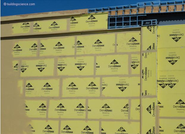
**Photograph 2: More New Systems** – Gypsum board sheets covered with trowel applied membrane.
