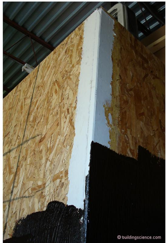
**Photograph 7: More Stress Reduction** - With outside corners we have more of a curve rather than a sharp change in direction.
