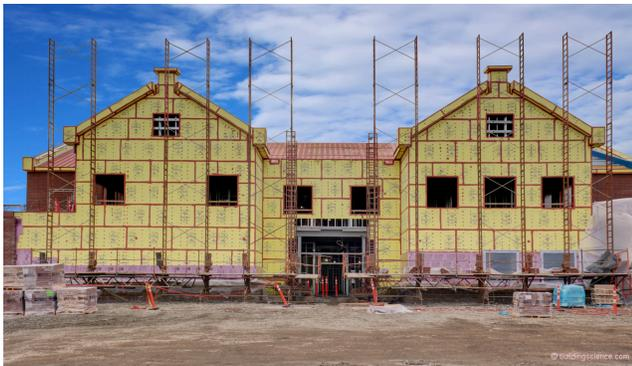
**Photograph 3: Still More New Systems** - Sheet goods with integral water and air control layers.
