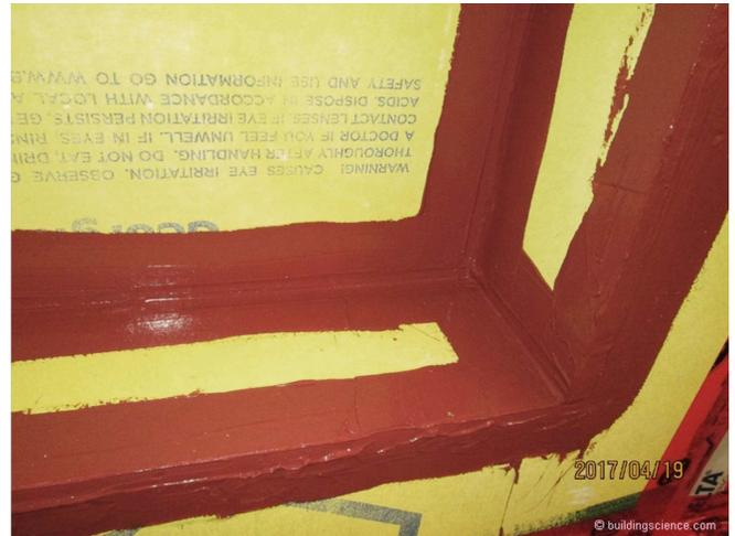
**Photograph 6: Stress Reduction** - So how to reduce the stress on the liquid applied membrane? Easy. Fill the joint with a sealant. Big improvement in performance. This works big time in corners. With inside corners a “fillet” bead yields a nice curve rather than sharp change in direction.
