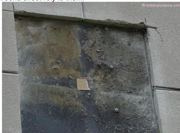
**Photograph 2: Stucco Bonded to Building Paper** - When stucco bonds to building paper the building paper loses water repellency and its' ability to drain.
