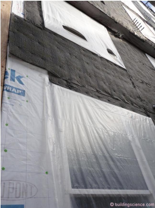
**Photograph 11: Drainage and Drying Gap** – Plastic wrap covered with a drainage mat with an integral bond break.
