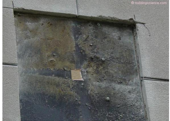
**Photograph 2: Stucco Bonded to Building Paper** - When stucco bonds to building paper the building paper loses water repellency and its' ability to drain.
