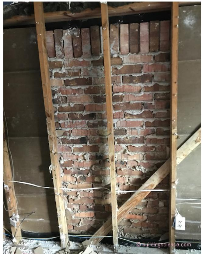
**Photograph 5: Backside of Brick** - Now it gets interesting...especially if you have brick. You cut away and get rid of all the interior gypsum board and cavity insulation and your sheathing leaving bare stud framing and naked exposed brick. When in doubt throw it out.
