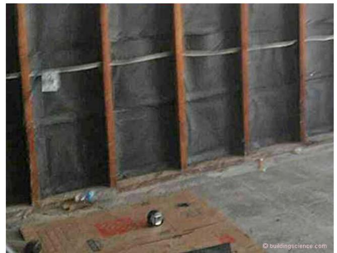
**Photograph 7: Drainage Mat –** The drainage mat is installed directly against the interior of the brick veneer...with the filter fabric facing inwards. Photograph courtesy of Joseph Pauwels.
