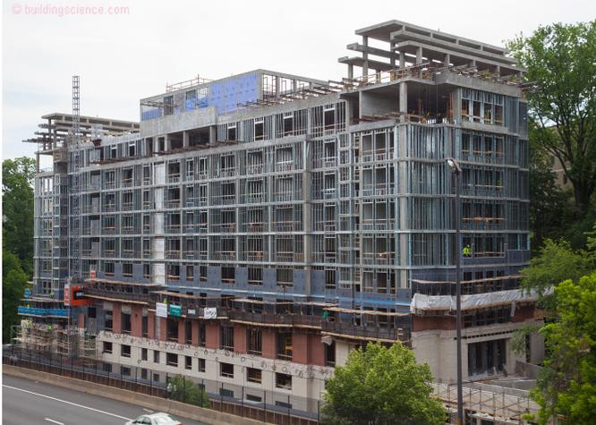
**Photograph 4: Multi-Story Concrete Frame Building - Steel-stud back-up walls with a non-combustible brick veneer cladding installed over a 1-inch air space. The sheathing is a direct applied (“to the steel studs”) foil-faced isocyanurate continuous insulation with sealed joints. This assembly has passed the NFPA 285 test. Replace the brick veneer with stucco, terracotta, cultured stone and metal panels and we would have similar results.**
