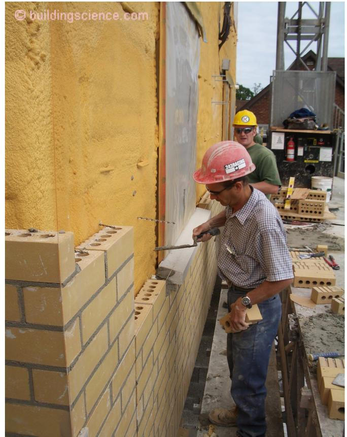
**Photograph 5: Mid-Rise Concrete Frame Building – Masonry back up wall with a 3-inch layer of 2 lb/ft<sup>3</sup> density spray polyurethane foam (SPF). The SPF is the continuous insulation layer – and is fire resistant but still combustible. The cladding is a non-combustible brick veneer over a ½ inch air space. This assembly has passed the NFPA 285 test.**
