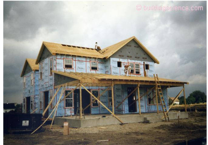
**Photograph 7: Low-Rise Wood Frame Building** - The continuous insulation layer is 1-inch extruded polystyrene insulation with sealed joints. The cladding (not installed) is direct applied vinyl siding. This assembly is not required to pass the NFPA 285 test.
