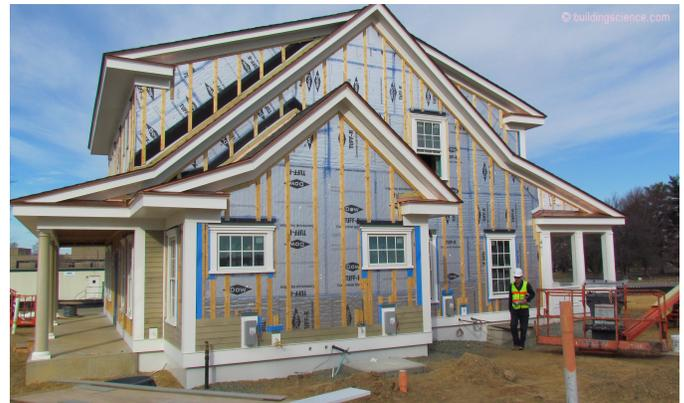
**Photograph 6: Low-Rise Wood Frame Building – This is the NIST Net Zero Energy Test House. The continuous insulation layer is 4 inches of foil-faced isocyanurate. The cladding is non-combustible fiber cement siding installed over 1x4 wood furring (¾-inch air space). This assembly is not required to pass the NFPA 285 test and would easily outperform the Grenfell Tower in a fire because of the fiber cement cladding and the small “rain screen” airspace (¾ inch)."**
