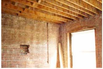
**Photograph 12: Typical Interior Condition** – To "parge or not to parge is the question..." Probably not necessary to apply the cementitious rendering here.
