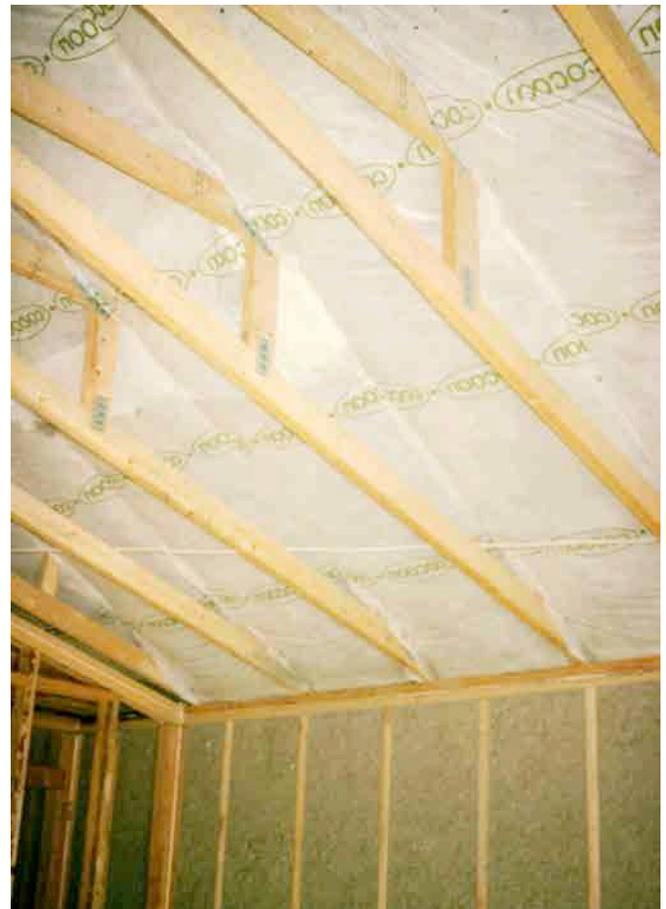
**Photograph 1: Flow-Through Assembly**—The most common insulation is netted cellulose although spray applied fiberglass, netted fiberglass and fiberglass batts are options.
