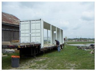
**Photograph 5: Adaptive Reuse** – The "building science research" version. This "test hut" was "anally" water and air sealed on the exterior and insulated on the interior with non water sensitive high-density (2 lb/ft<sup>3</sup>) spray polyurethane foam (SPF). Minimum of 2 inches of SPF yields a vapor transmission of less than 1 perm. You get a Class II vapor retarder, which means you can use this approach everywhere – even in Tuktoyaktuk.
