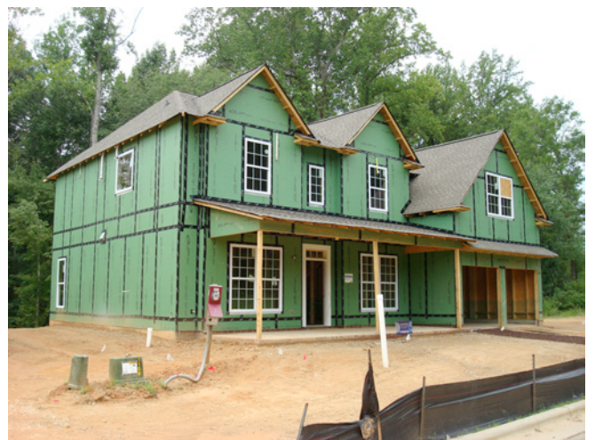
Photograph 1: OSB Water Control Layer – OSB where the water control layer is integral with the OSB sheathing where taping the joints provides water control layer continuity.
