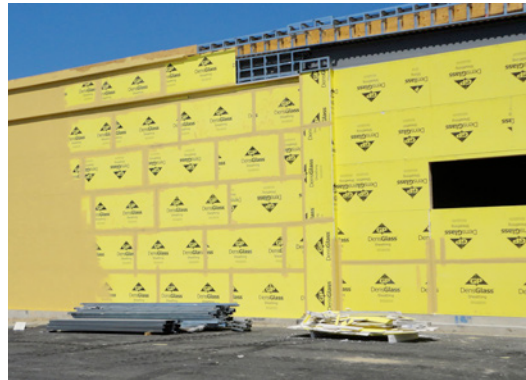
Photograph 5: Fully Adhered Membrane (above left) - In commercial and institutional buildings fully adhered membranes are the “gold standard.” But it took 20 years. These are now true “peel and stick” systems when primers are used. Photograph 6: Liquid Applied Membrane (above right) - Becoming common now. Note the joint treatment – a tape reinforced mastic is installed at the joints first – then over coated with a liquid applied membrane creating as seamless, jointless system.
