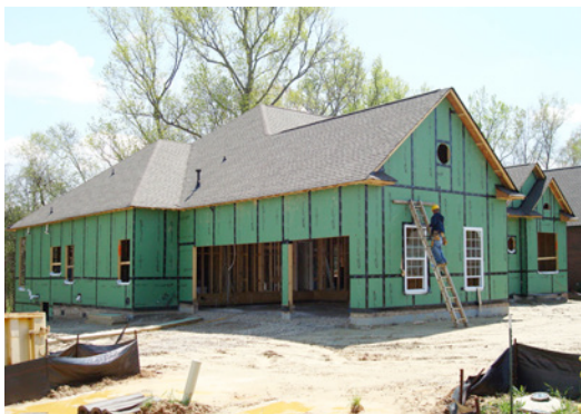
Photograph 8: Wood Sheathing (above left) - Residentially we now use tapes on wood sheathings that have factory applied membranes factory bonded to them to provide water management and air management. Photograph 9: Foam Sheathing (above right) - Foam plastic sheathing panels are taped together creating a water-resistive barrier system. These systems are now around 20 years old. This image dates back to a subdivision development in Chicago in 1995. 3M was one of the first to develop acrylic based tape system for housewraps in the 1980's and they migrated to foam sheathings in the 1990's.
