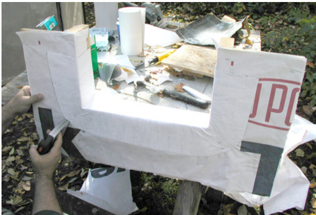
Photograph 3: Formable Flashing (above left) – Life got better when flashing systems became formable and flexible. This photo dates back a decade to when I got my first sample of flexible flashing to play with in my back yard. I thought it was the greatest invention since the transistor. Ok, so I am exaggerating - but only a little. Look at how beautifully a seamless under window flashing system is created. Photograph 4: No Origami Here (above right) – Today’s liquid applied systems easily handle complex geometries seamlessly.
