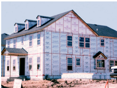
Photograph 8: Wood Sheathing (above left) - Residentially we now use tapes on wood sheathings that have factory applied membranes factory bonded to them to provide water management and air management. Photograph 9: Foam Sheathing (above right) - Foam plastic sheathing panels are taped together creating a water-resistive barrier system. These systems are now around 20 years old. This image dates back to a subdivision development in Chicago in 1995. 3M was one of the first to develop acrylic based tape system for housewraps in the 1980's and they migrated to foam sheathings in the 1990's.
