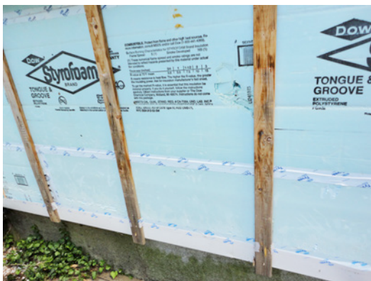
Photograph 8: Wood Sheathing (above left) - Residentially we now use tapes on wood sheathings that have factory applied membranes factory bonded to them to provide water management and air management. Photograph 9: Foam Sheathing (above right) - Foam plastic sheathing panels are taped together creating a water-resistive barrier system. These systems are now around 20 years old. This image dates back to a subdivision development in Chicago in 1995. 3M was one of the first to develop acrylic based tape system for housewraps in the 1980's and they migrated to foam sheathings in the 1990's.
