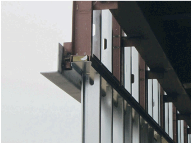
Photograph 5: Stand-Off - Can be welded to plates cast into slabs or welded to structural steel supports.
