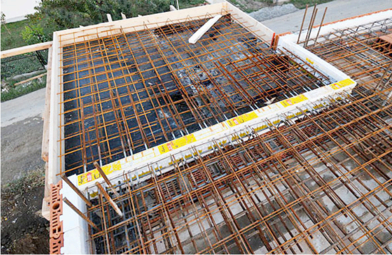
Photograph 3: Belgrade Balcony – Nice view of the Danube River from a thermally broken balcony. OK, the river is out there somewhere. I have not been to Serbia recently, but apparently they can afford more efficiency than Chicago. It can't be the climate because Chicago is much colder in the winter. The real estate values must be really something in Belgrade compared to Chicago. Good thing in Chicago we have green roofs. Don't seem to be many of those in Belgrade either. Priorities are important. The R-value of dirt apparently does not impress Serbs. Image courtesy of Beodom, Inc., Belgrade, Serbia.
