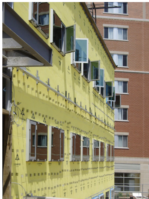
Photograph 7: A Little Bit of Everything - Relieving angles on stand-offs and bumped out windows. Nice. Wonder if there are any LEED points for this? Yeah, probably not.
