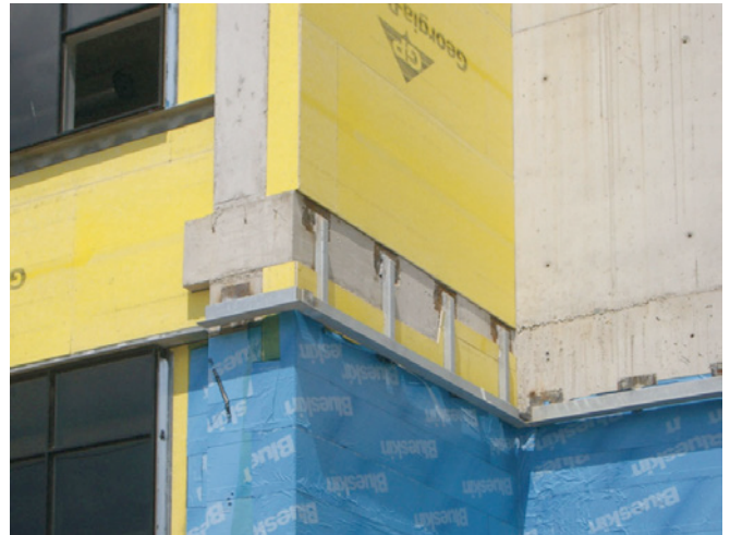
Photograph 6: Relieving Angle Line Up – Notice how the relieving angle lines up with the top of the window bringing joy to The Architect. Clever, elegant and simple structural engineering. Hope the structural engineer got lunch out of this one.
