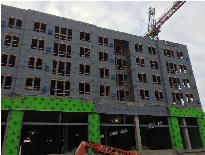
**Photograph 1 – Multi-Story Gypsum Sheathing:** Typical “podium” construction. Exterior vapor open gypsum sheathing covered with a “sweet spot” water resistive barrier (wrub) or building paper or building wrap or water control layer – between 10 and 20 perms.
