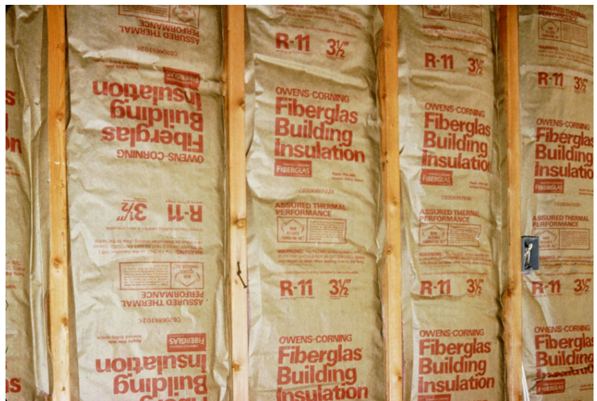
Photograph 1: Kraft-Faced Batt —Humble and ubiquitous with a dry cup value of 1 perm so it meets the code requirement of a Class II vapor retarder as tested under ASTM E-96 Test Method A (the desiccant method). Its wet cup value is around 10 perms.
