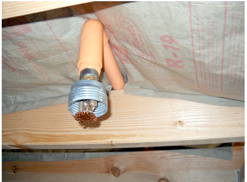
Photograph 3: Tenting —Many “authorities having jurisdiction” insist that sprinklers and the sprinkler lines have insulation only installed above them – no insulation under them – and that they be inspected with the insulation in place before gypsum board is installed. The only practical way to do this is by “tenting” kraft faced batts over them. Don't forget to blow loose fill insulation over the “tentted” batt insulation. Photograph courtesy of Steven Winter Associates.
