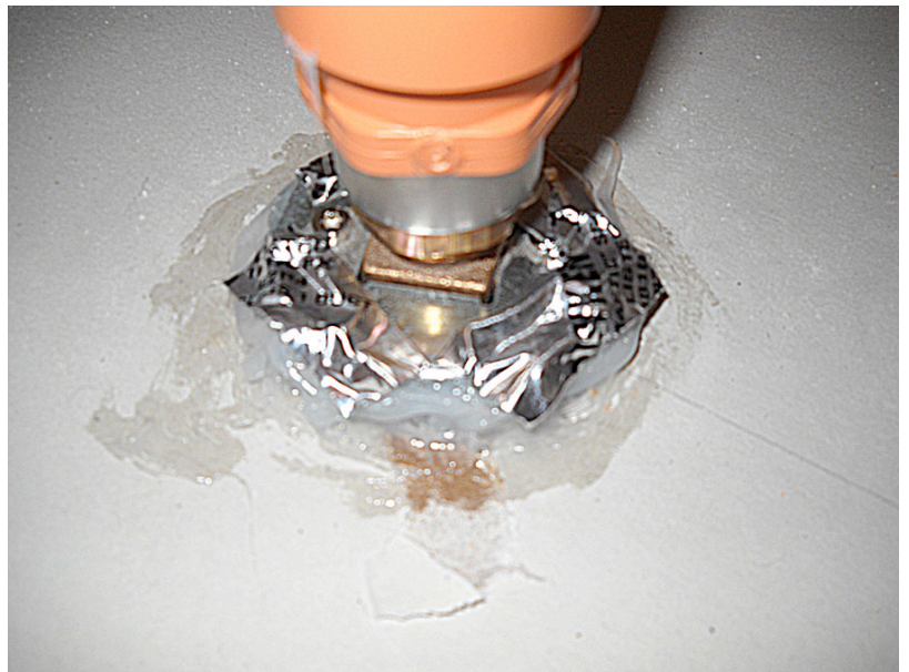
Photograph 4: Big Holes — Sprinkler heads and escutcheon plates need to be airtight where they penetrate the ceiling. The problem is have they been tested in this configuration?
