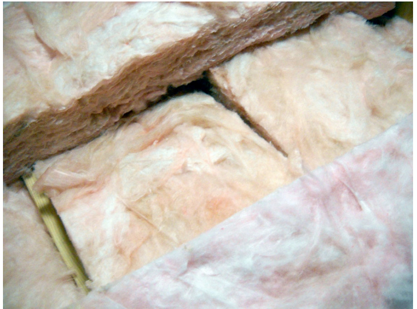
Photograph 2: Mind the Gap —Batts don't fit very well in horizontal applications. Blow loose insulation over the top of them – use blown fiberglass or blown cellulose. Guess what we call it? Batt and blow. Photograph courtesy of Steven Winter Associates.
